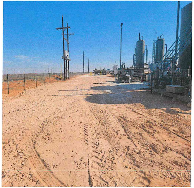
Backfill to grade and compacted pad, view east.
