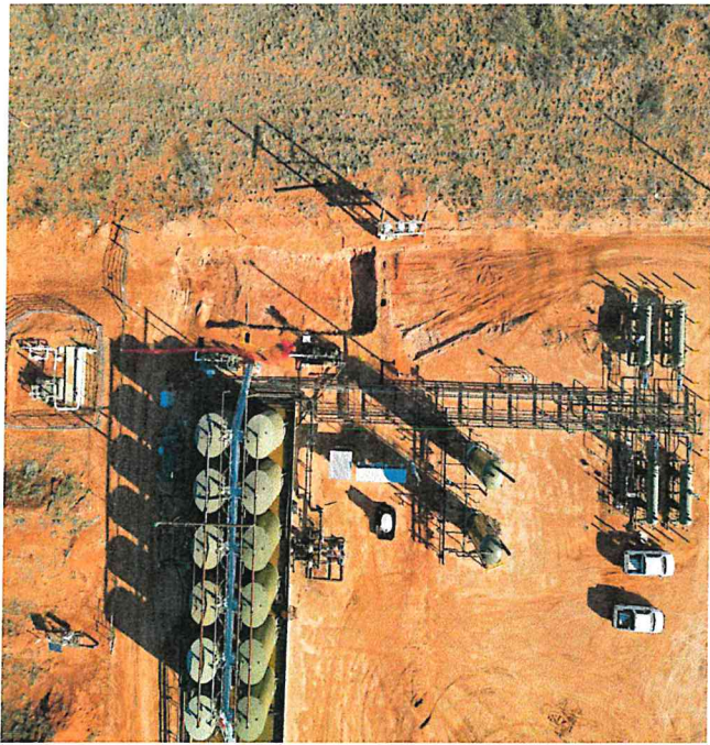
Aerial of excavation.
