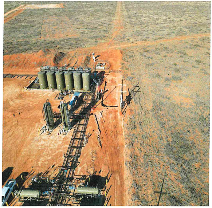
Aerial of Excavation.
