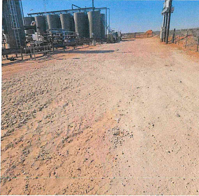
Backfill to grade and compacted pad, view west.
