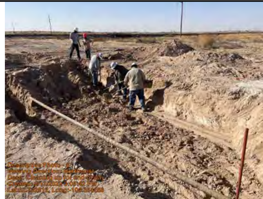
Shovel Work Around Pipelines
