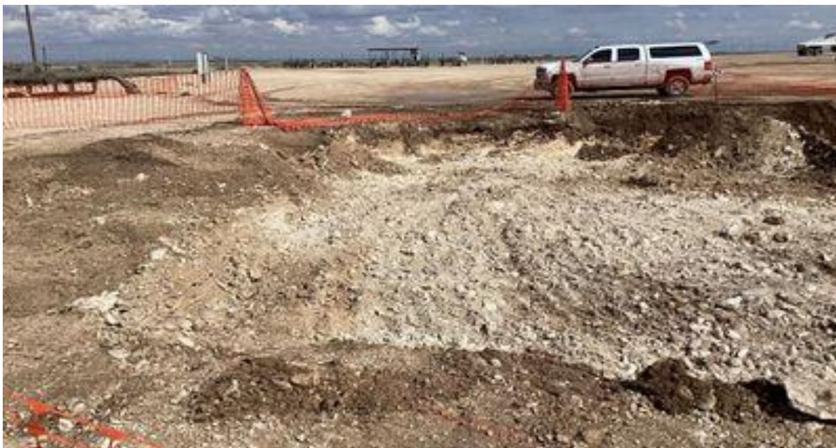
Photo 3 View Looking North - Remedial Over-Excavation.
