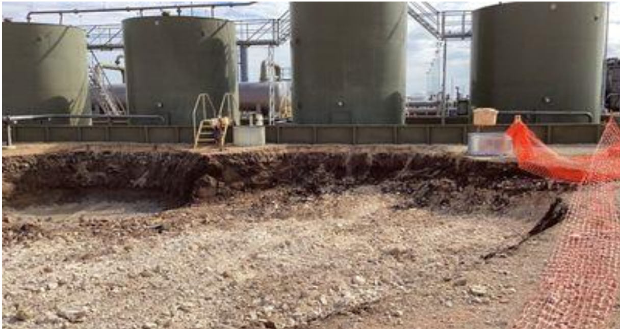
Photo 1 View Looking East - Remedial Over-Excavation.
