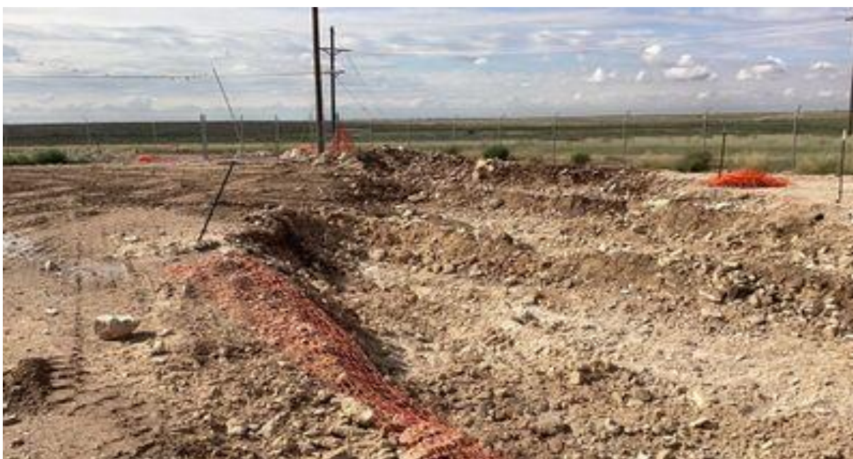
Photo 4 View Looking South - Remedial Over-Excavation.
