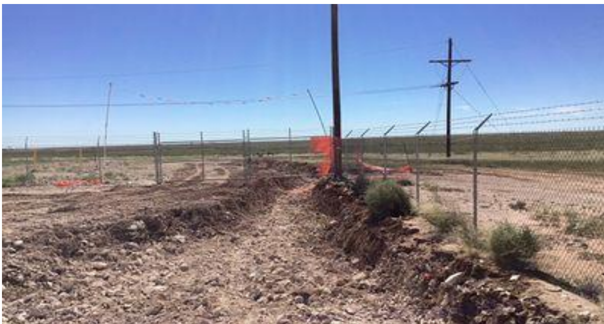
Photo 8 View Looking South - Excavation.
