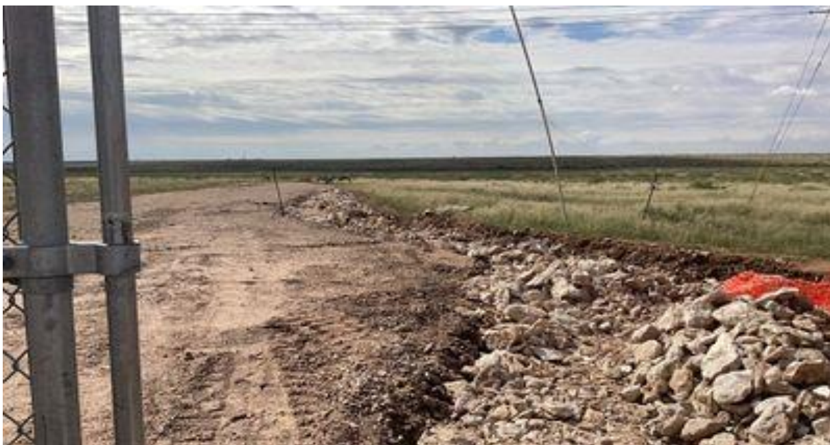
Photo 6 View Looking South - Remedial Over-Excavation - Material Pending Removal.
