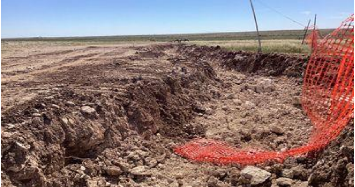
Photo 9 View Looking South - Excavation.
