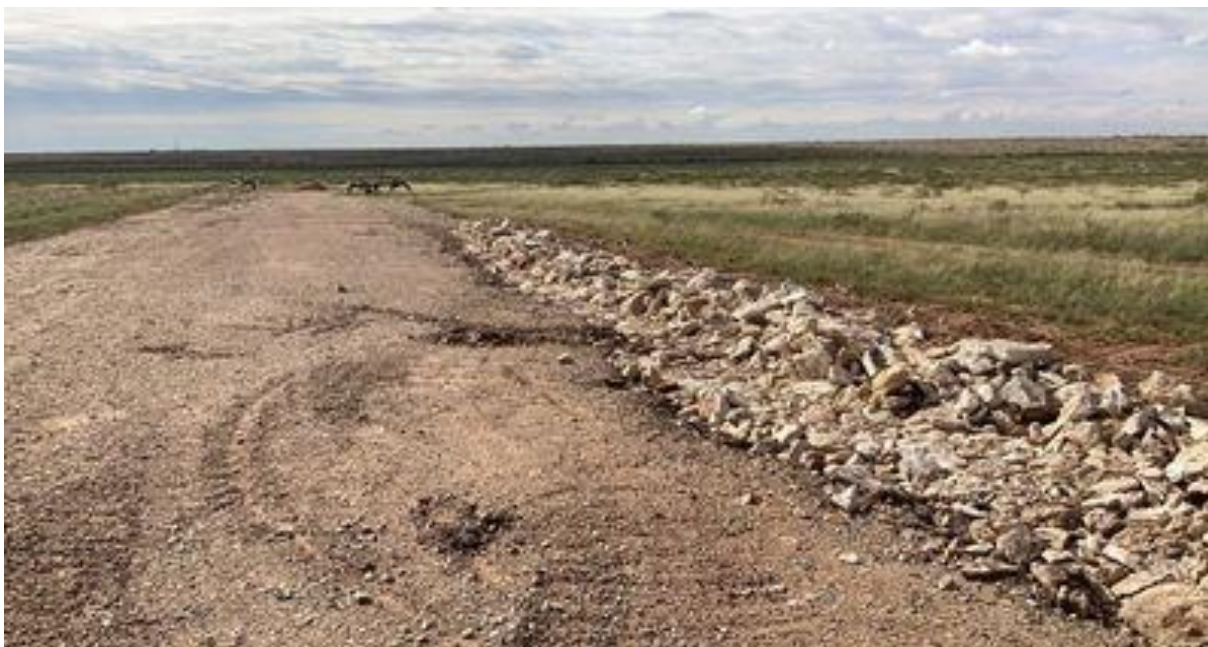
Photo 7 Remedial Over-Excavation - Material Pending Removal.
