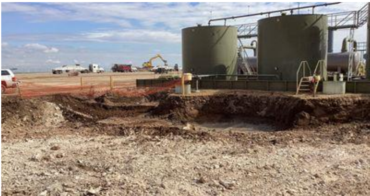
Photo 2 View Looking North - Remedial Over-Excavation.
