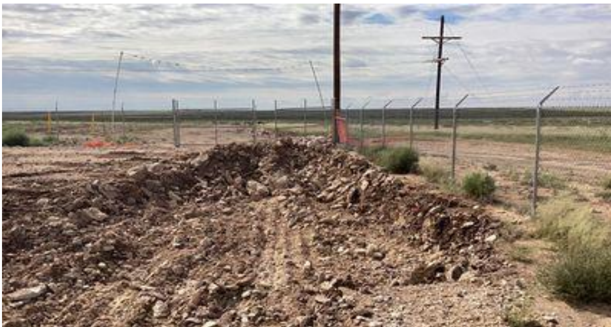
Photo 5 View Looking South - Remedial Over-Excavation.
