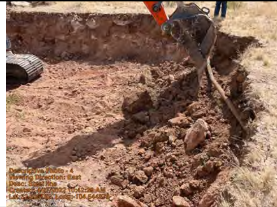
Steel line about 50' south of berm. Called Michael Jordan who reported that the line has been purged and we can continue digging around it
