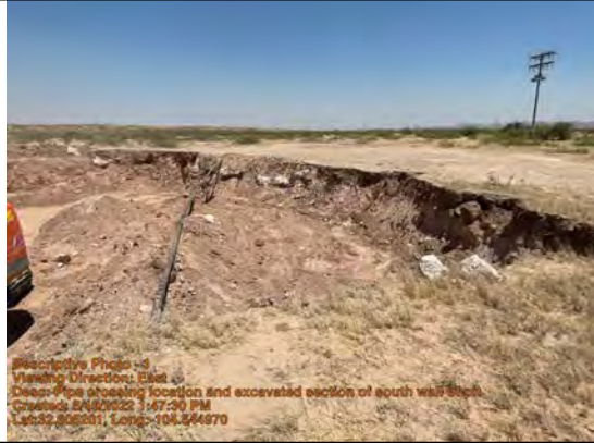
Pipe crossing location and excavated section of south wall of pit
