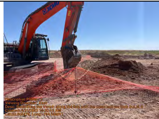
Backfilling the trench along the line with the clean soil we took out of it
