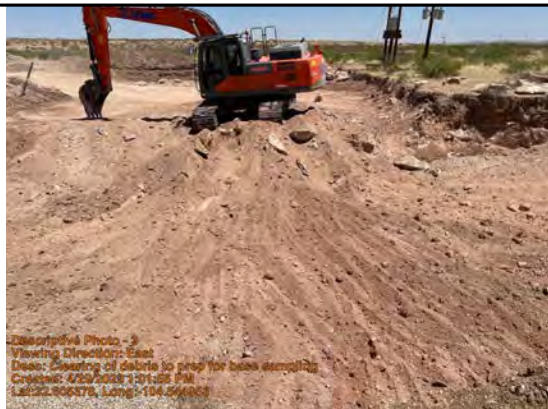
Clearing of large rock debris to prep for base sampling
