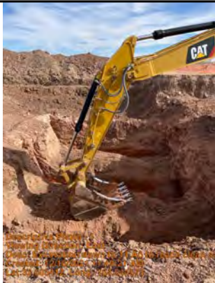
Excavation down to 14' to reach clean sample
