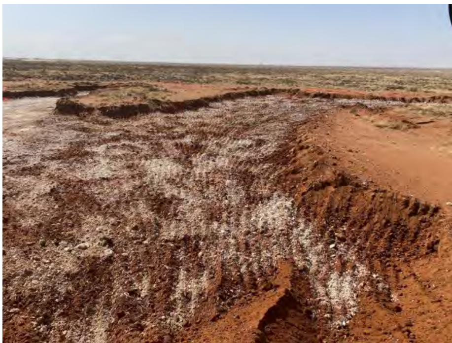
Figure 1: Excavation continues throughout the contaminated area until excavation sampling confirms extent of plume.
