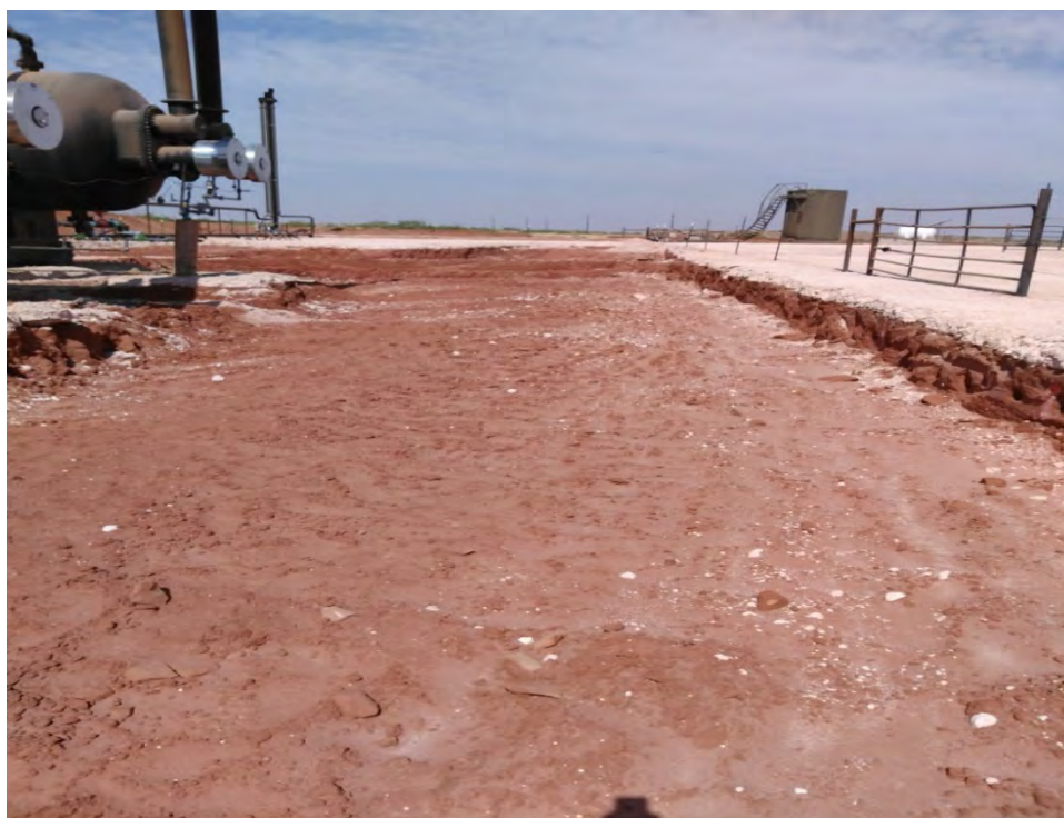
Photo 18: West-facing view from the central part of the excavation showing the western margin of the excavation in the background.
