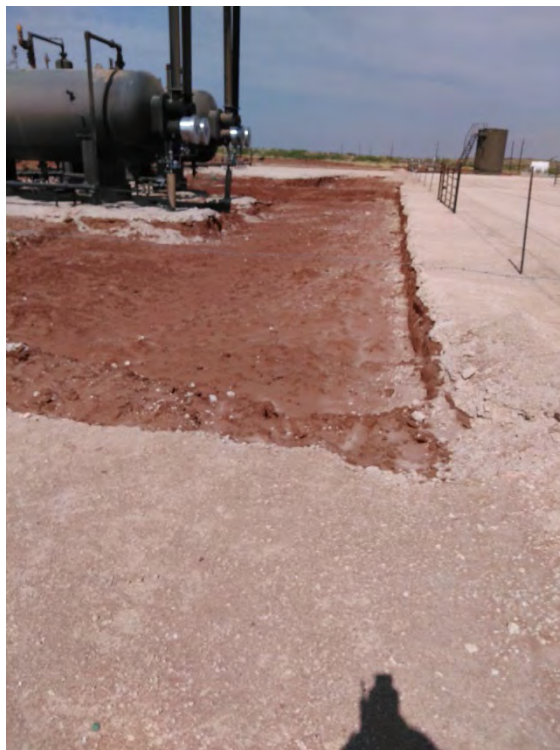
Photo 17: West-facing view of the eastern (foreground) and northern (right) margins of the excavation.
