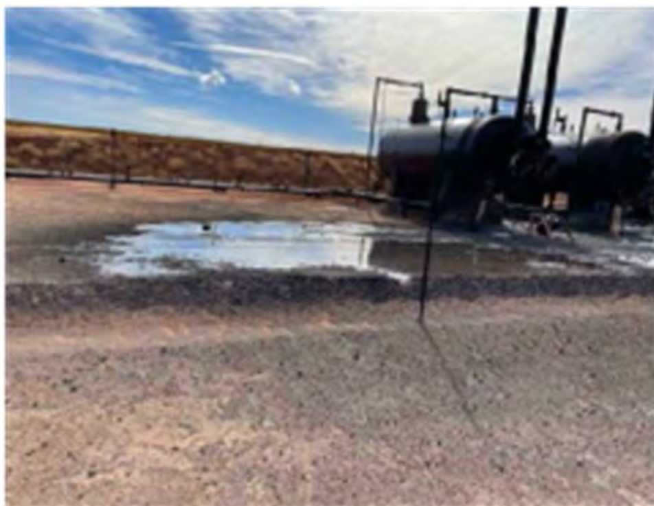
Photo 6: View of free liquids within the containment area at east end of release area facing south-southwest.
