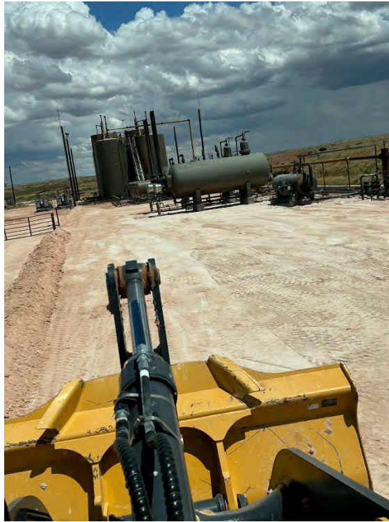
Photo 33: East view showing completed backfill of excavation, repaired CTB berm and replaced gate.
