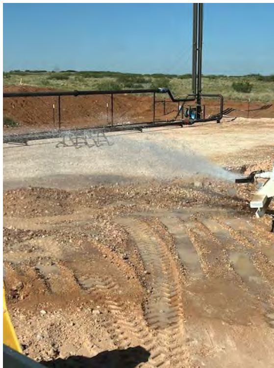
Photo 30: Southeast view of watering during compaction of backfill near the gas flare.
