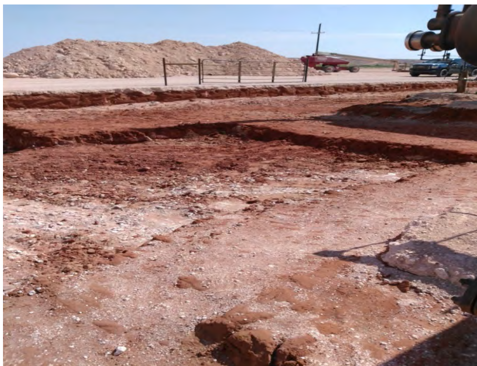
Photo 22: View of excavated area facing northeast
