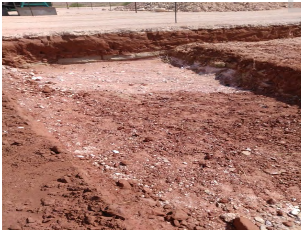
Photo 23: View of excavation facing north-northeast showing the northern end of the buried flowline buffer area on the right.
