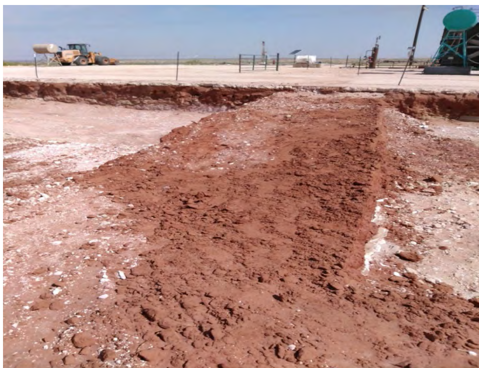
Photo 24: North-facing view of the buried flowline buffer area. This area was scraped to shallow depth to protect buried flow lines running north to the compressor station in the background.
