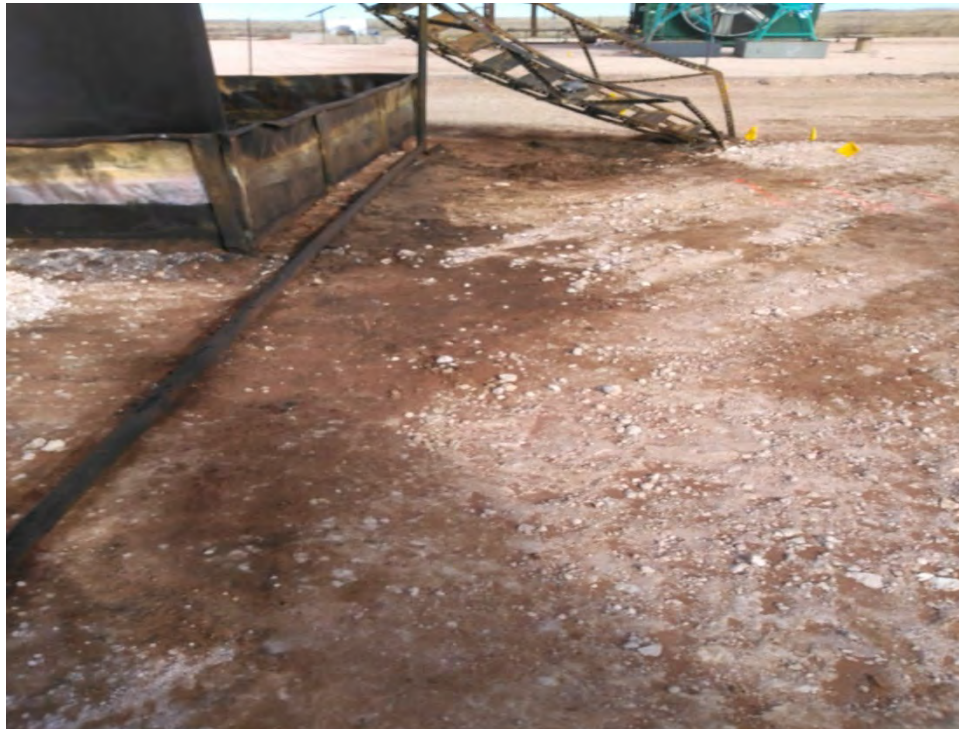
Photo 10: View of release area staining on east side of day tank containment facing north.
