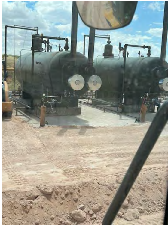
Photo 29: South-southeast view of backfill material at separators.
