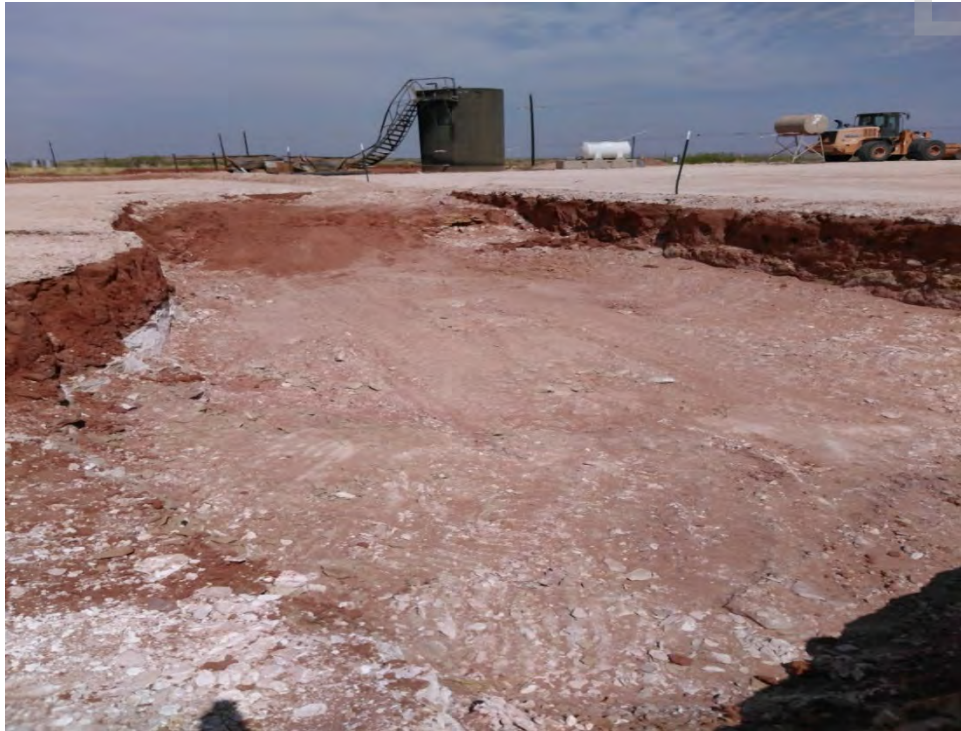
Photo 27: View of excavated area's western boundary facing west-northwest.
