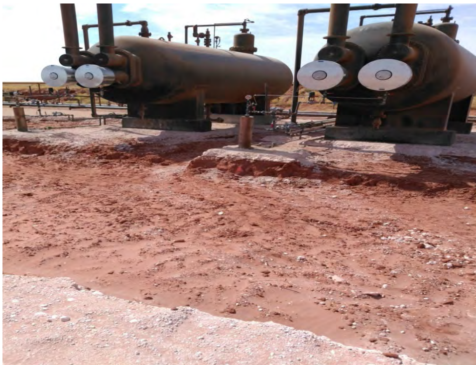
Photo 20: View of excavated area north of vessels facing southeast.
