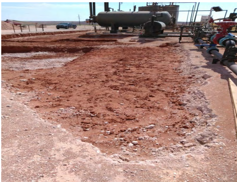
Photo 26: East-facing view of excavated area along flare piping.
