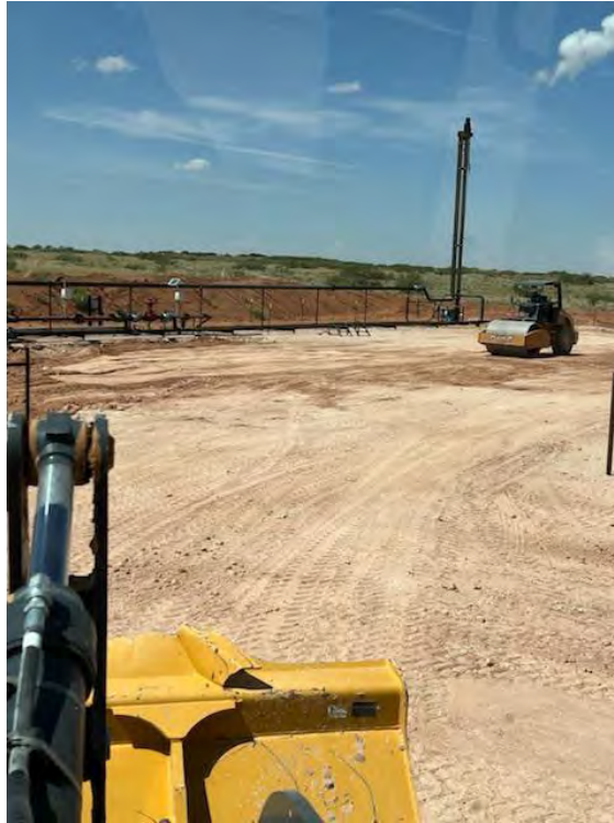
Photo 31: Southeast view of compaction of backfill near the gas flare.
