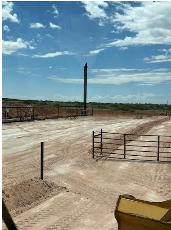
Photo 32: Southeast view of completed backfill. Note facility berm has been repaired and facility gate replaced.
