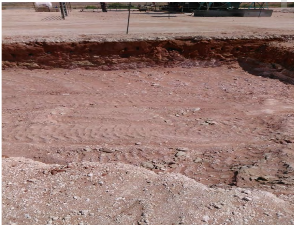
Photo 25: View of excavated area west of buffer area facing north-northeast.
