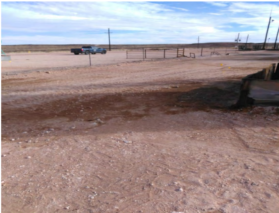
Photo 8: View of release area staining facing northeast.
