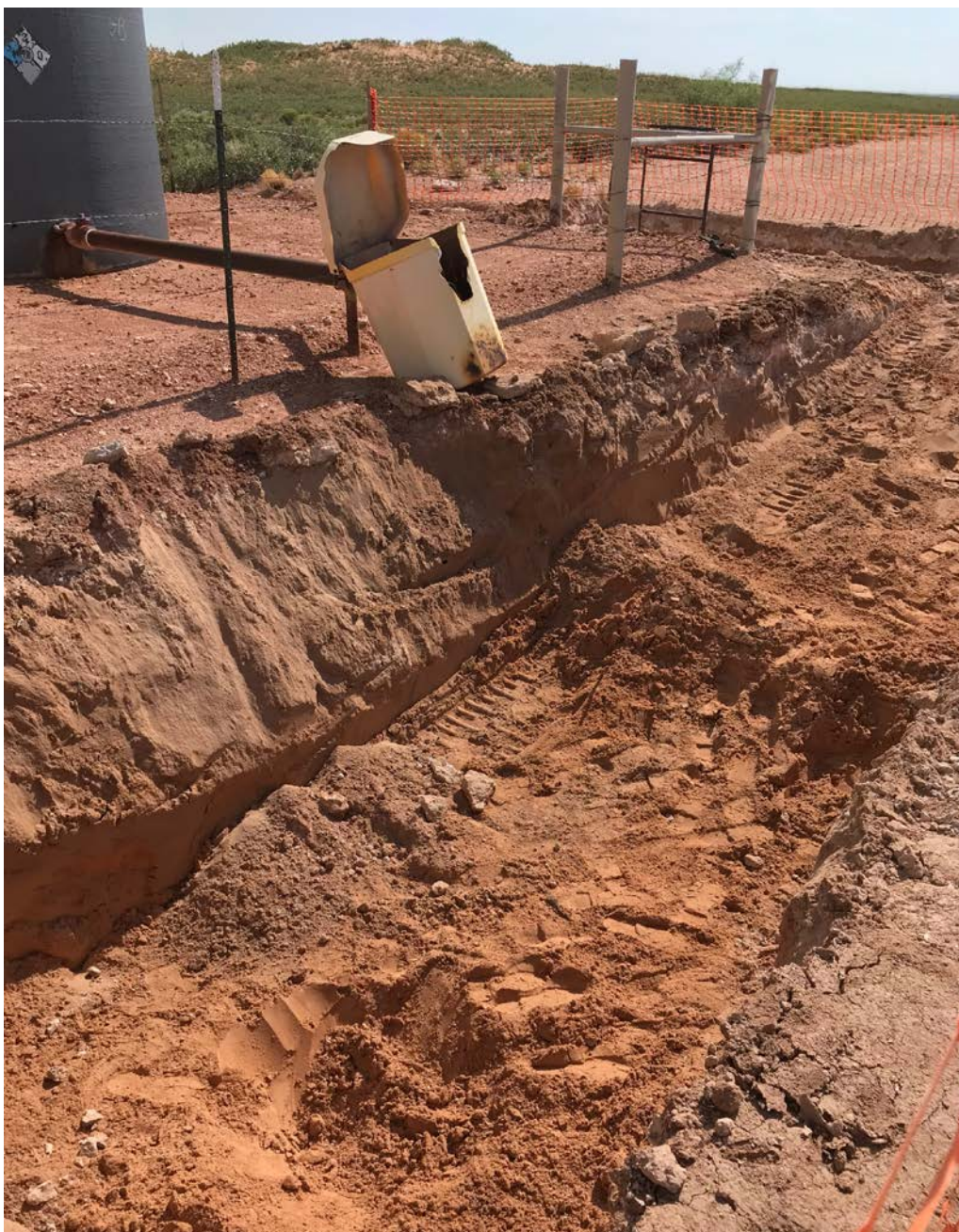
Southwest facing view of the open excavations.
