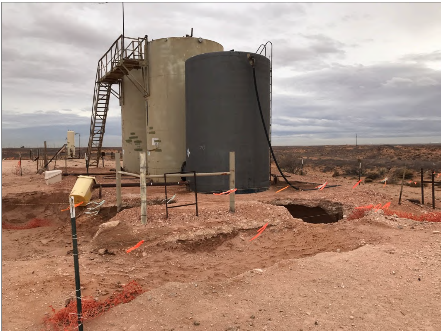
East facing view of the open excavations.
