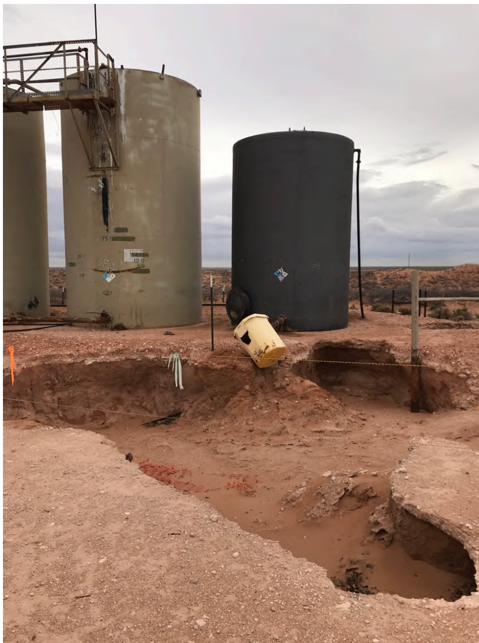
South facing view of the open excavations.
