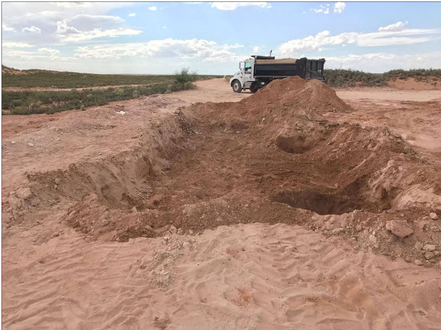
West facing view of the open excavations, post tank removal.
