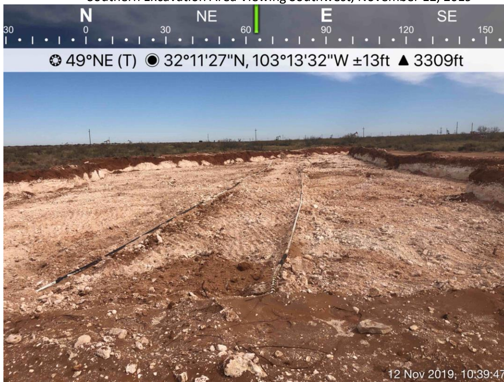
Southern Excavation Area Viewing Northeast, November 12, 2019
