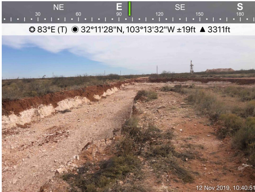
Southern Excavation Area Viewing East, November 12, 2019
