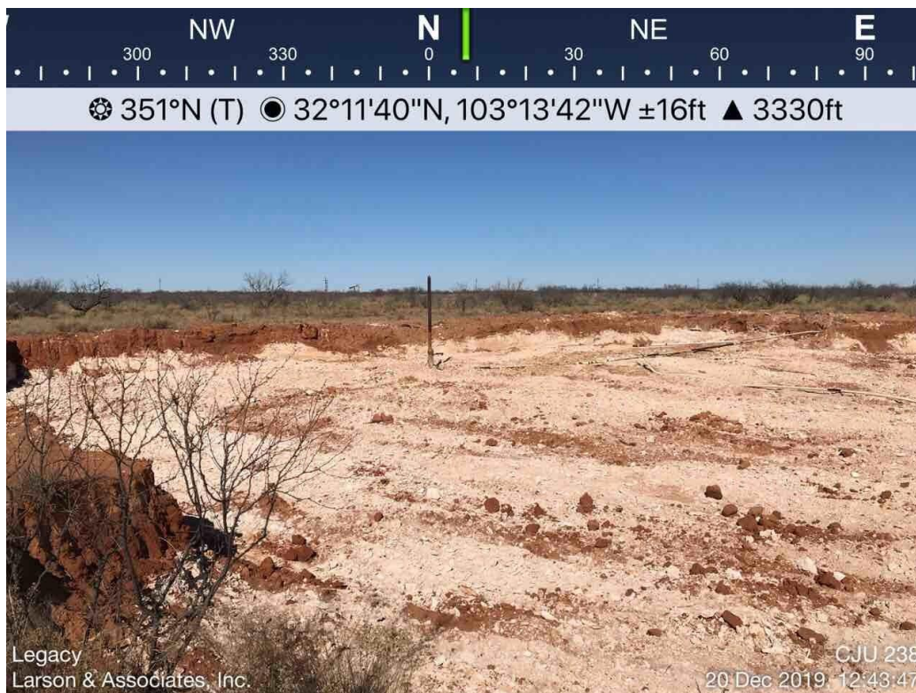
Northern Excavation Area Viewing Northwest, December 20, 2019
