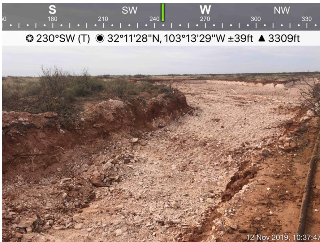
Southern Excavation Area Viewing Southwest, November 12, 2019
