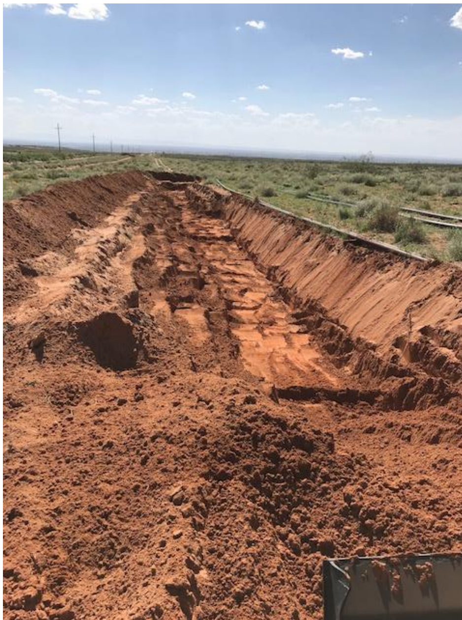
Photograph 2: View west of excavation.
