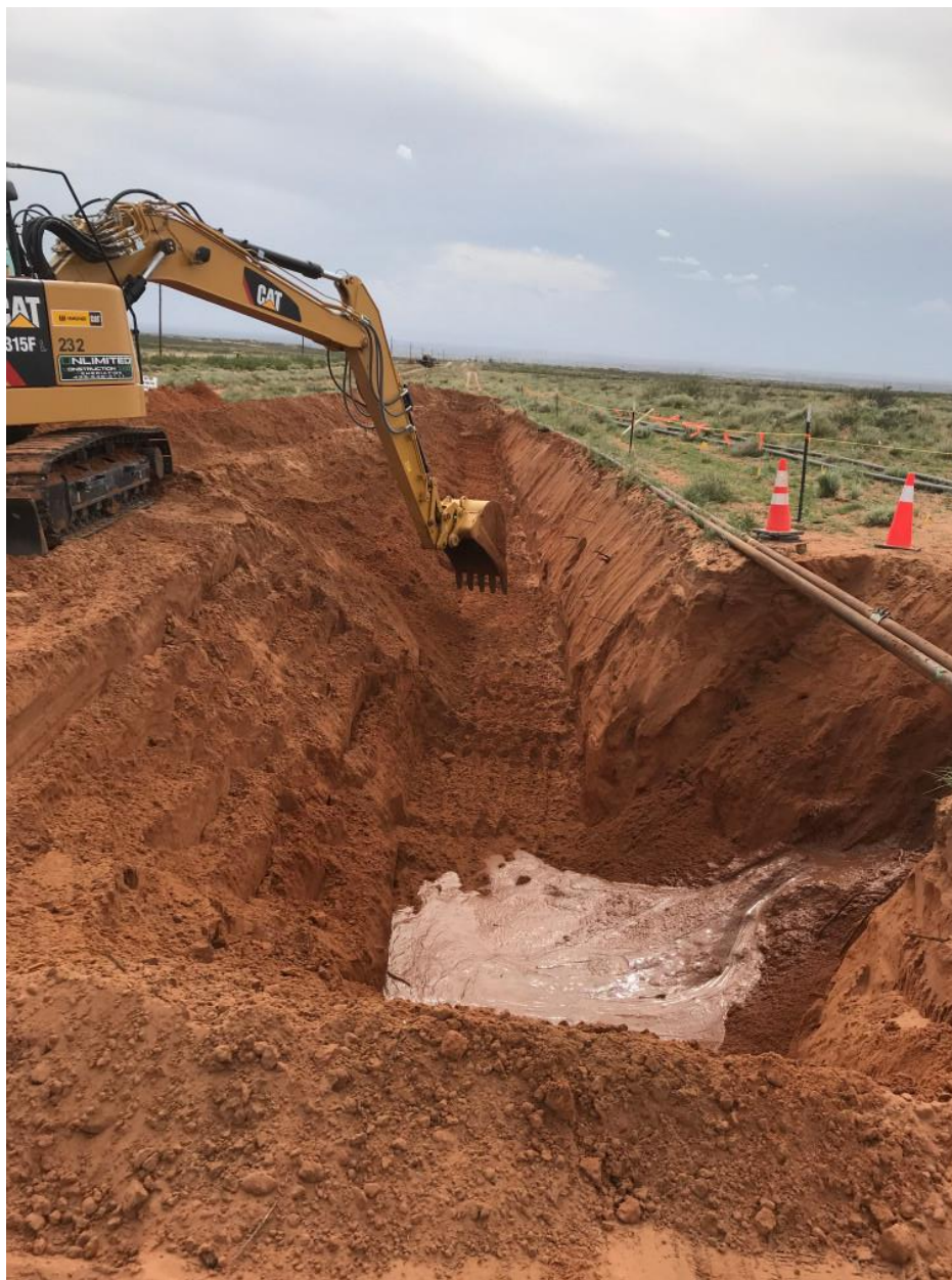
Photograph 1: View east of excavation.
