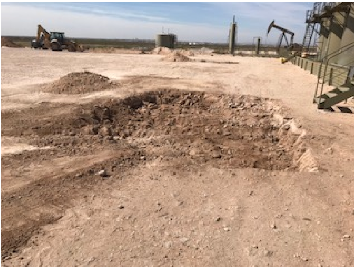
Excavation in area of SS02 – view west
