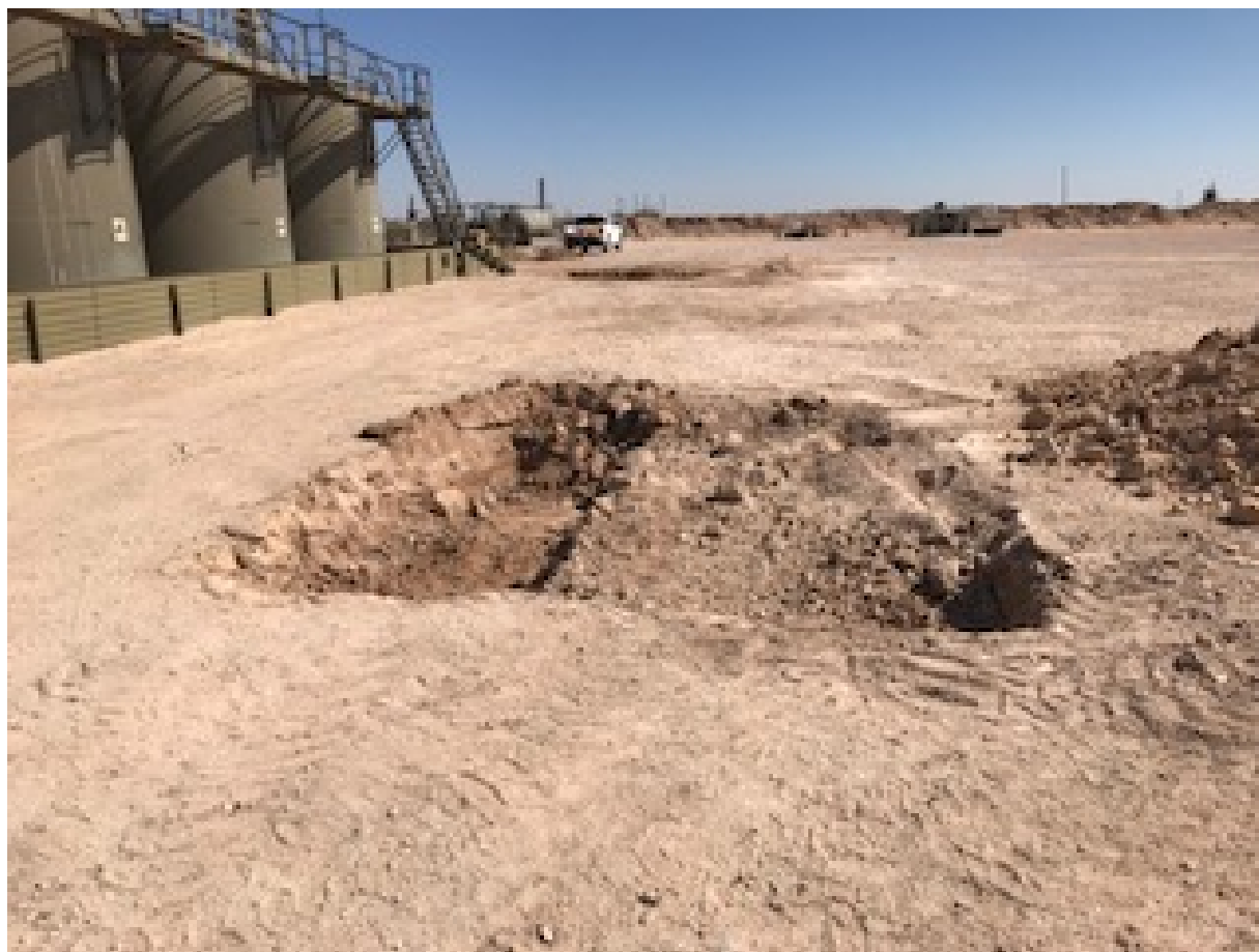
Excavation in area of SS01 – view northeast
