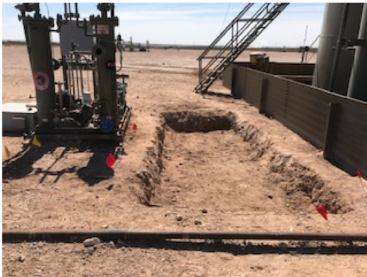
Excavation in area of SS03 – view south
