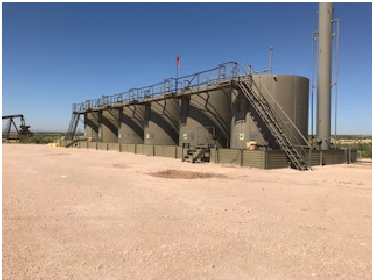
Release footprint on pad surface before excavation– view northwest.
