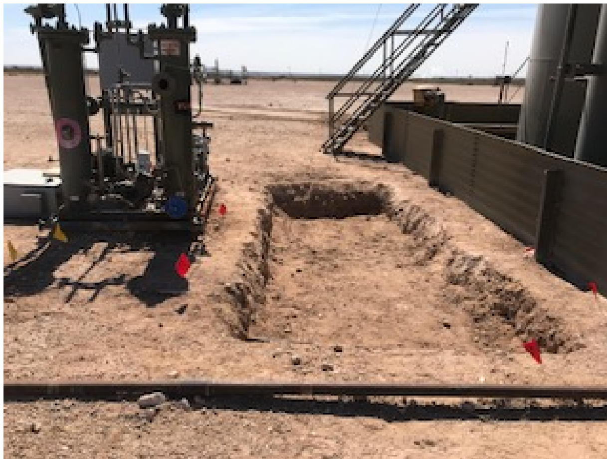
Excavation in area of SS03 – view south
