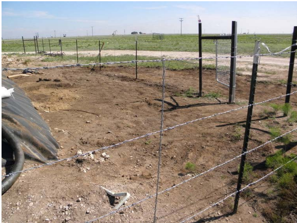
Photo 4 – View of impacted soil remediation activity facing north-northeast
