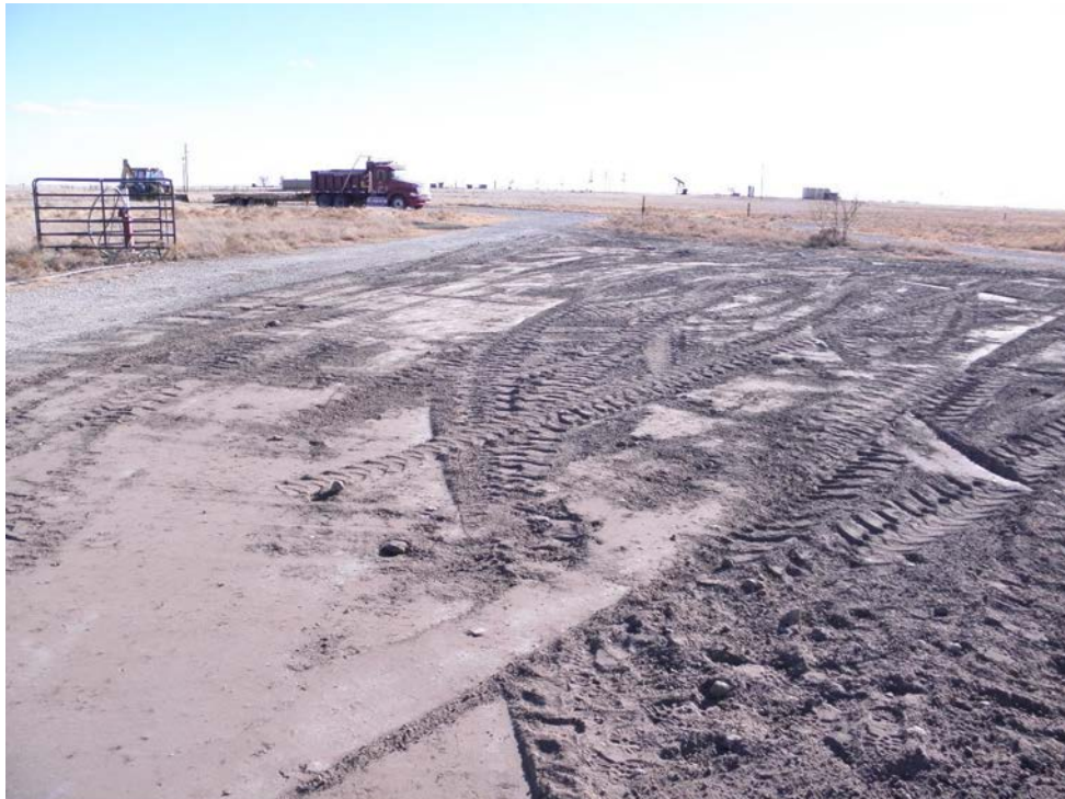
Photo 8 – View of backfilled excavated area south of AST facing south
