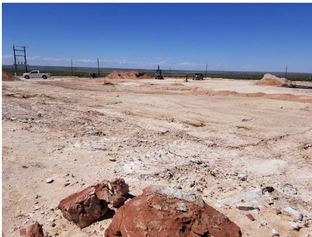
Backfilling excavated areas
