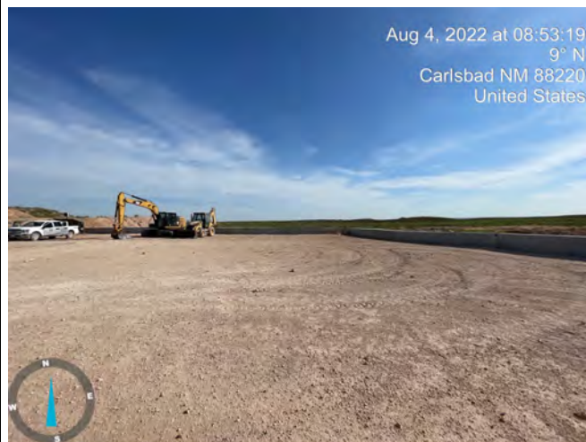
Photograph: 1 Date: 8/4/2023 Description: Excavation preparation View: North
