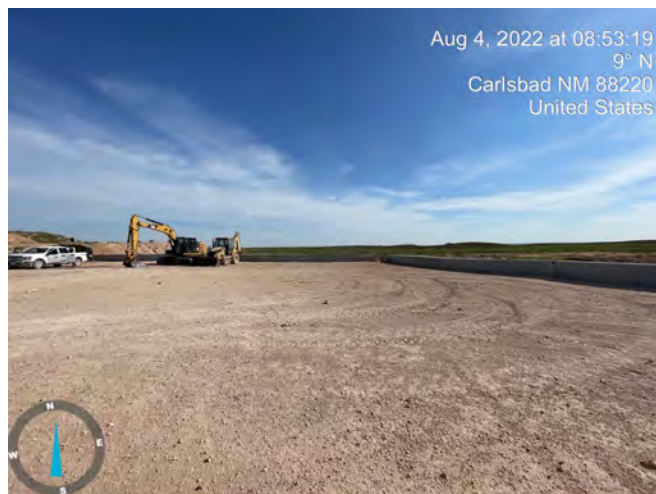
Photograph: 1 Date: 8/4/2023 Description: Excavation preparation View: North
