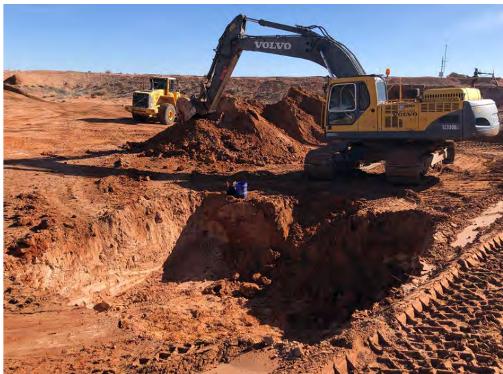
Figure 4: Remediation at SWB-02 to 5-feet below containment base. Photo is viewing northeast from SWW-03. 32.4201972, -103.6041028. 2023-02-23.
