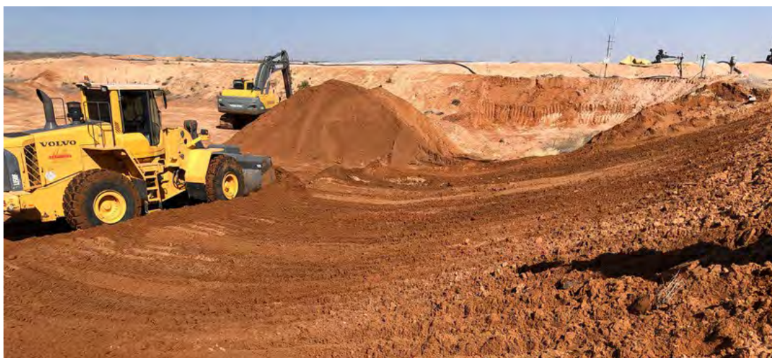
Figure 3: Remediation at the southwest corner. Photo viewing east from the southwest corner of containment. The southeast corner remediation is visible in photo background-right. Stockpiled soil is being hauled off-site for proper disposal. Date: 02/23/2023. GPS: 32.4201500, -103.6040556.
