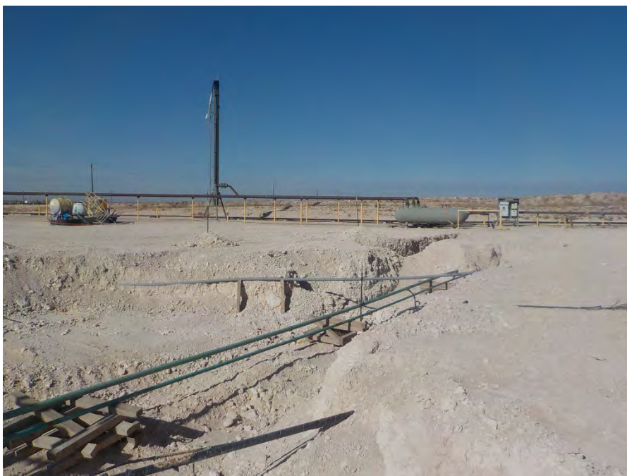
View of assessment and excavation activities at the site on March 29, 2022. Excavation around the site wellhead, view is towards the west.
