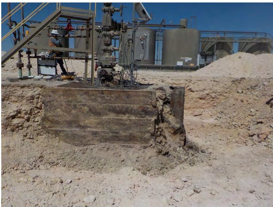
View of assessment and excavation activities at the site from March 7 through March 11, 2022. Excavation around the site wellhead, view is towards the north.
