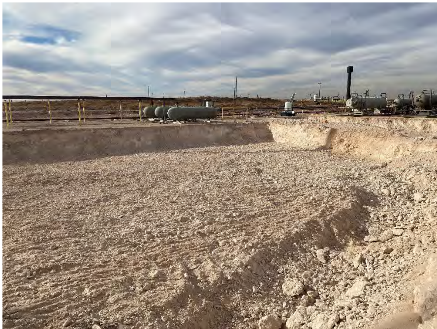
View of Ex-3 observed at the site on December 1, 2021. View is towards the west.
