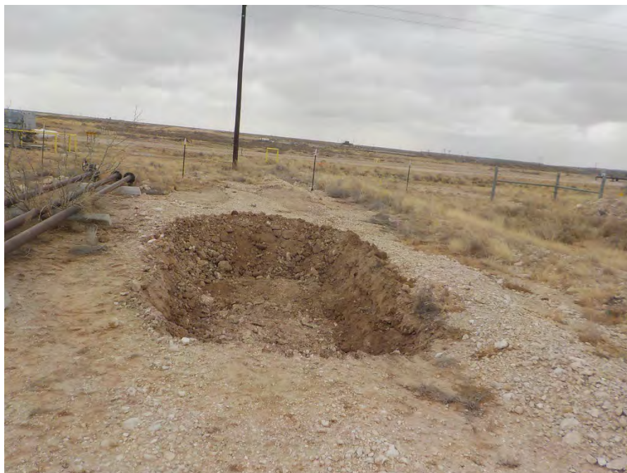
View of assessment and excavation activities at the site from March 7 through March 11, 2022. Excavation around the C-3 area, view is towards the south.
