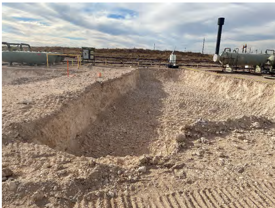
View of Ex-4 observed at the site on December 1, 2021. View is towards the west.
