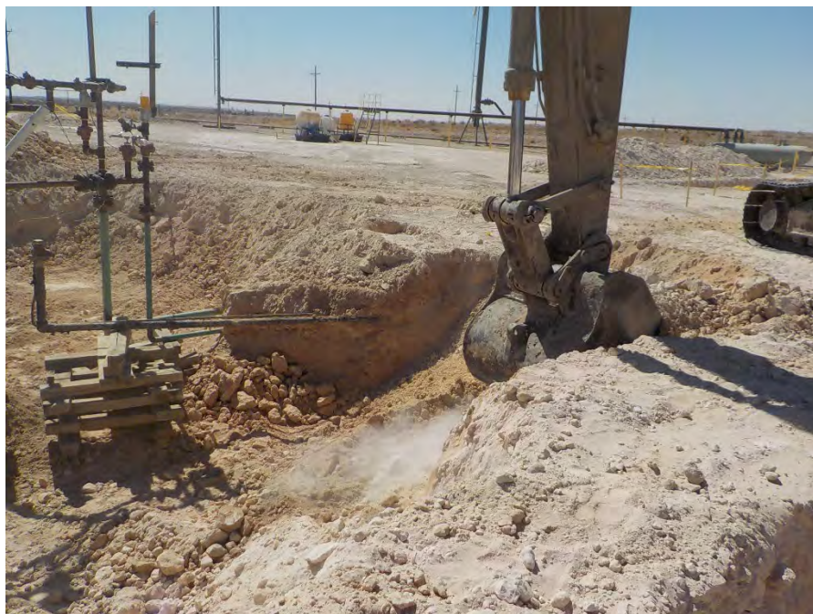
View of assessment and excavation activities at the site from March 7 through March 11, 2022. Excavation around the site wellhead, view is towards the west.
