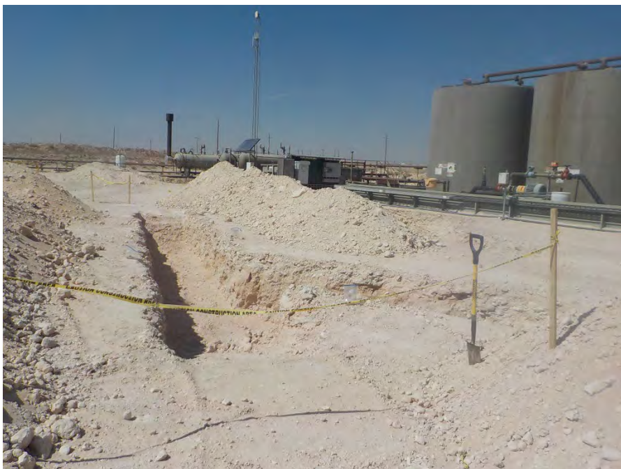
View of assessment and excavation activities at the site from March 7 through March 11, 2022. View is towards the west-northwest.
