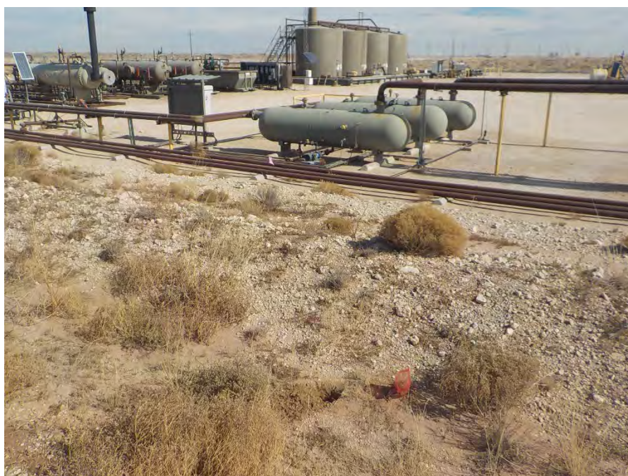
View is of surface sample SS-Northwest on January 14, 2022. View is towards the east.
