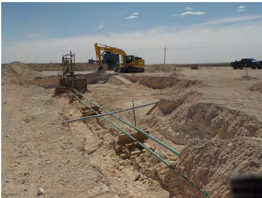
View of assessment and excavation activities at the site on March 29, 2022. Excavation around the site wellhead, view is towards the east.
