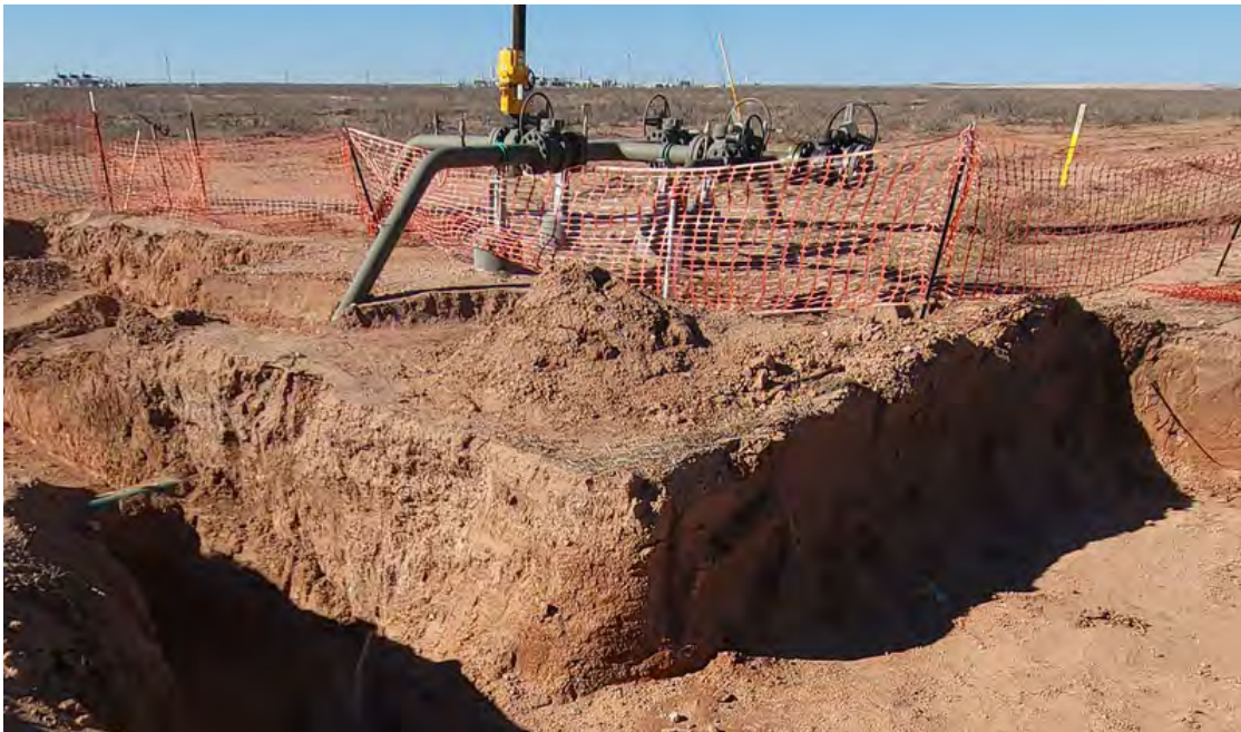
Figure 6: Excavation around south riser. Photo is viewing northwest. 2023-01-26 14:30:23. GPS: 32.1098390 N, 103.2798130 W.
