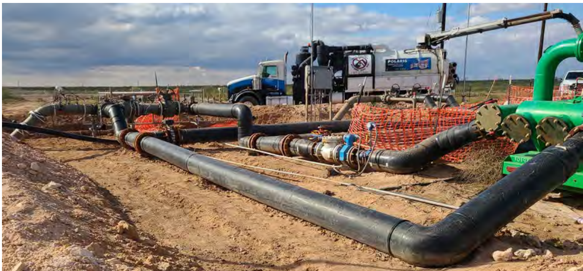
Figure 4: Hydrovac'ing around pipeline risers, at source, to remove mass load of impacted material. Photo is viewing southwest. 2022-10-28 15:07:26. GPS: 32.1113517 N, 103.2796717 W.
