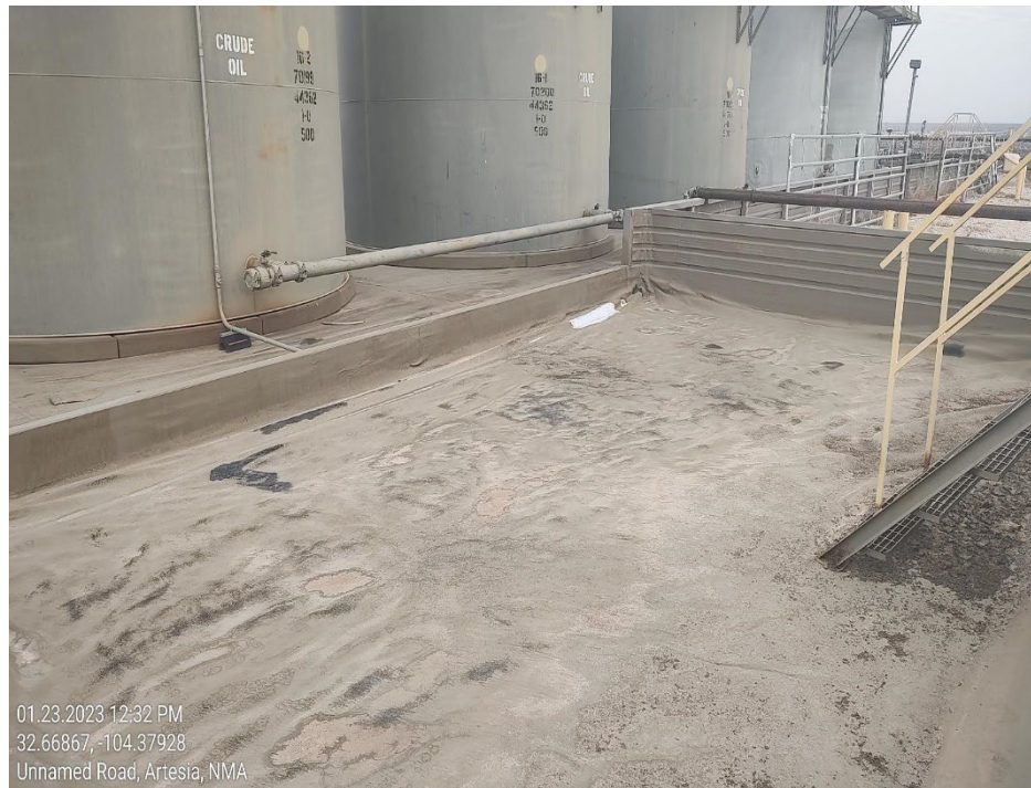
PHOTO 5: CTB Overflow Containment Liner NE
