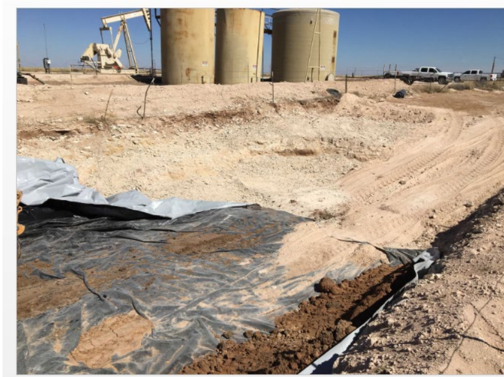
View of excavation/lining of 1RP-4891 facing northeast.
