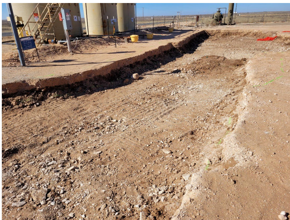
View of excavation facing west.
