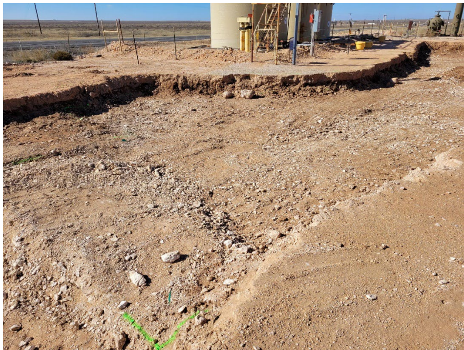
View of excavation facing west.
