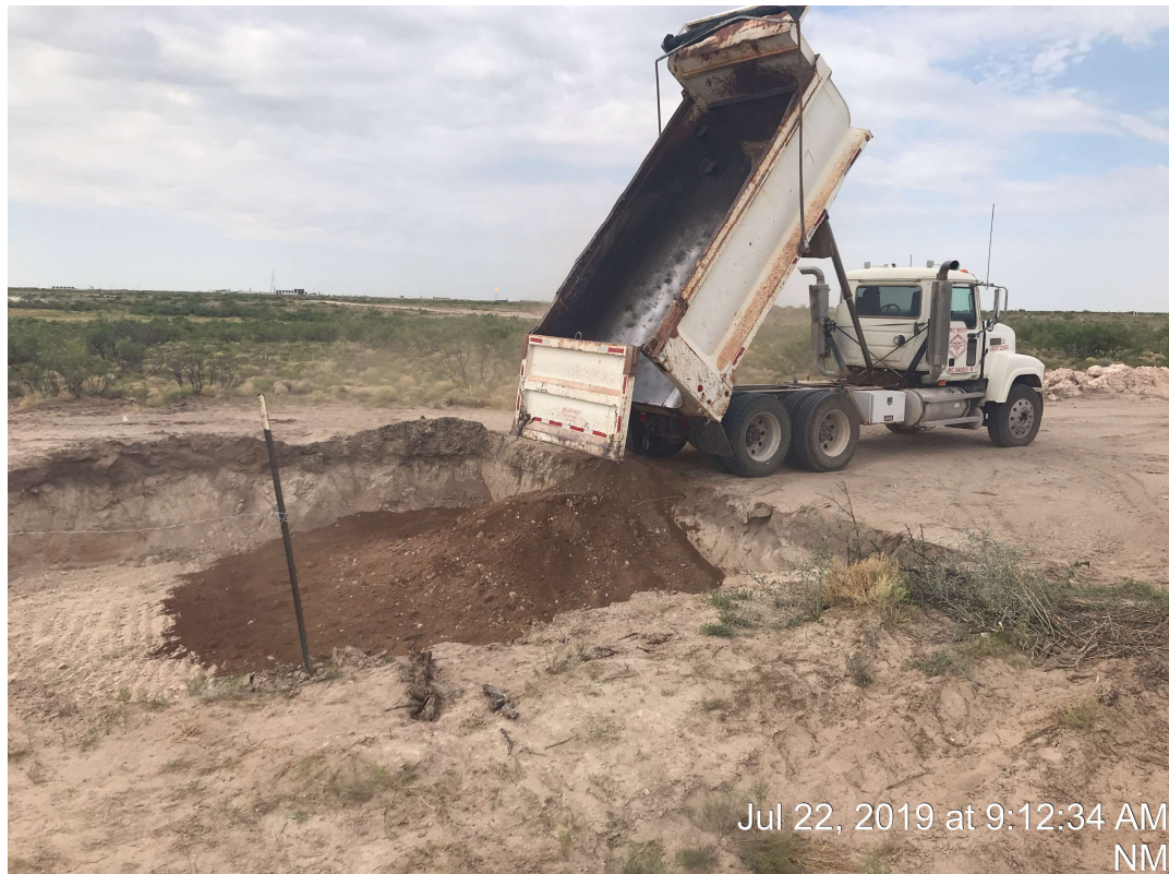
View of the backfilling of the northern excavated area.
