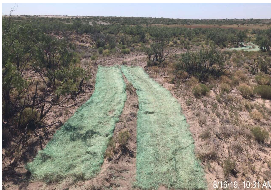
View of the remediation activities (placement of erosion control blanket and boulders) .
