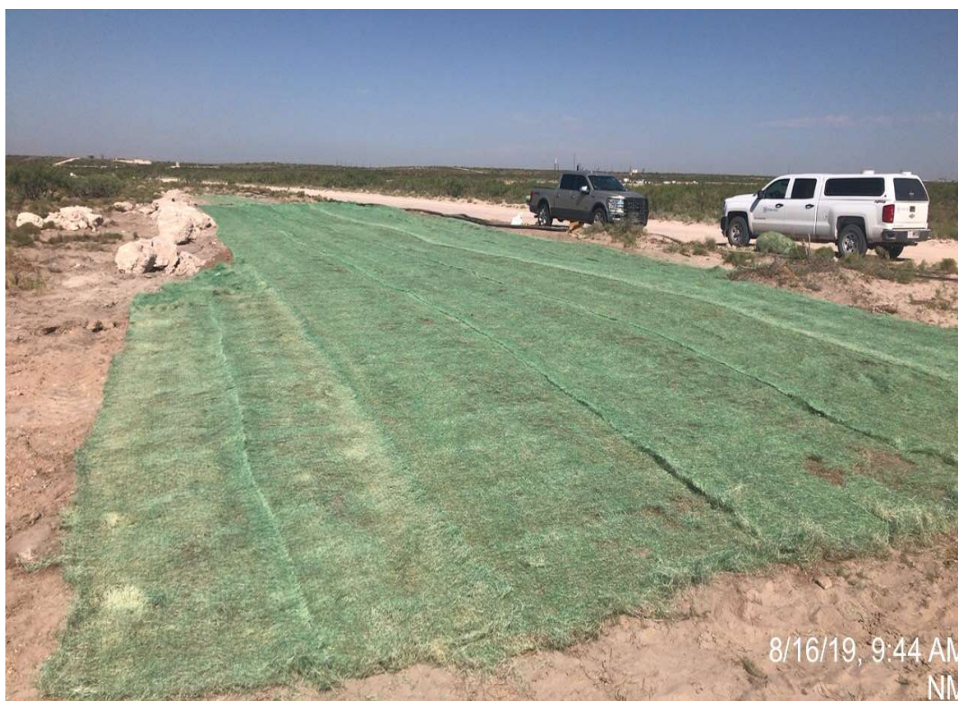
View of the remediation activities (placement of erosion control blanket and boulders) .
