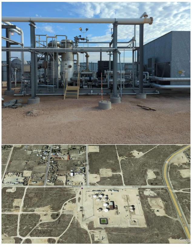
Compressor went down on high lube oil feed temperature. Due to ambient temperature of 105 degrees. The lube oil temperature became too hot.
