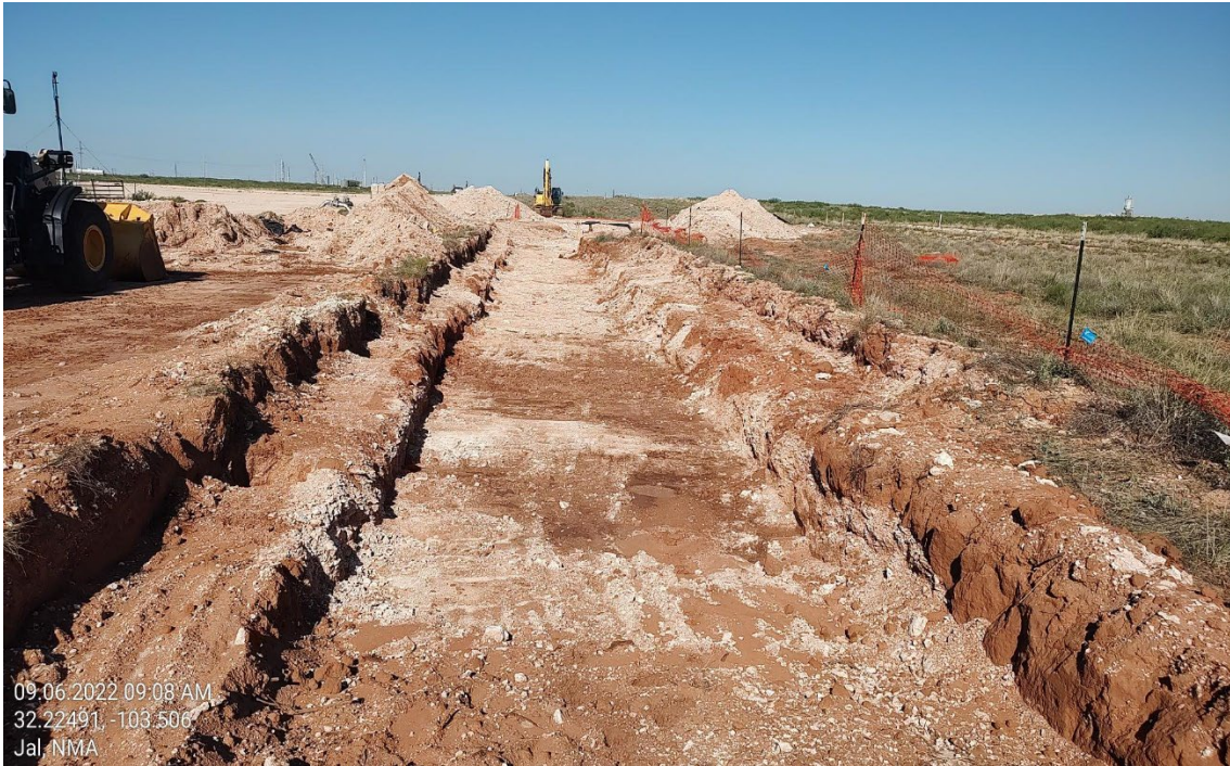
PHOTO 3: View of excavation, facing West / GPS: 32.22491, -103.506
