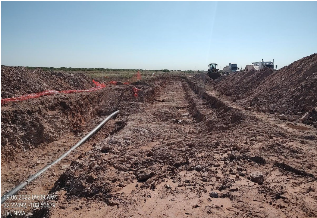
PHOTO 2: View of excavation, facing East / GPS: 32.22492, -103.50679
