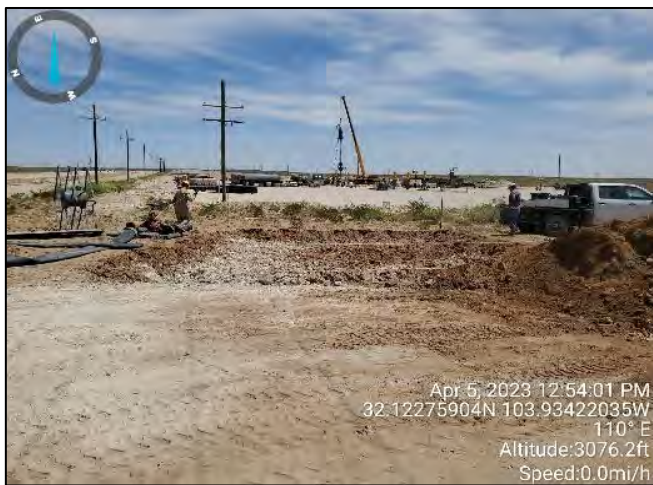
Photograph: 4 Date: 4/5/2023 Description: Excavation Activities View: East
