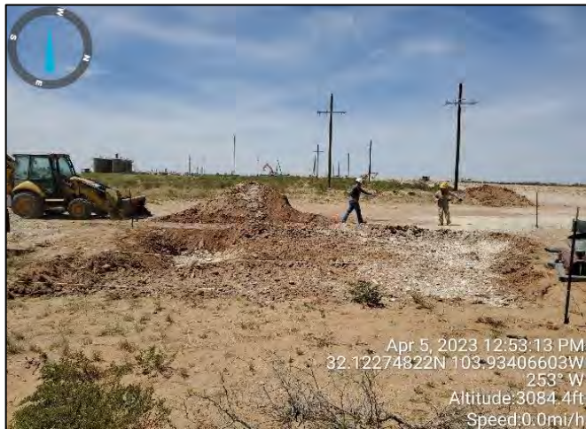
Photograph: 3 Date: 4/5/2023 Description: Excavation Activities View: West
