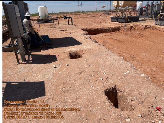
Hydrovaccated lines to be backfilled.
