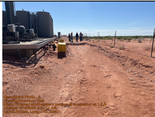
Finished southeastern portion of excavation at 1.5'.
