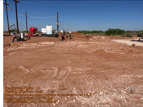
Finished southern portion of excavation at 1.5'.
