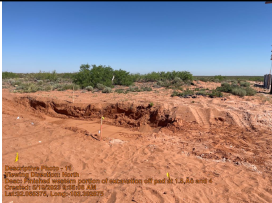
Finished western portion of excavation off pad at 1.5' and 4'.
