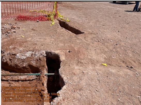
Hydrovaccated lines to be filled.
