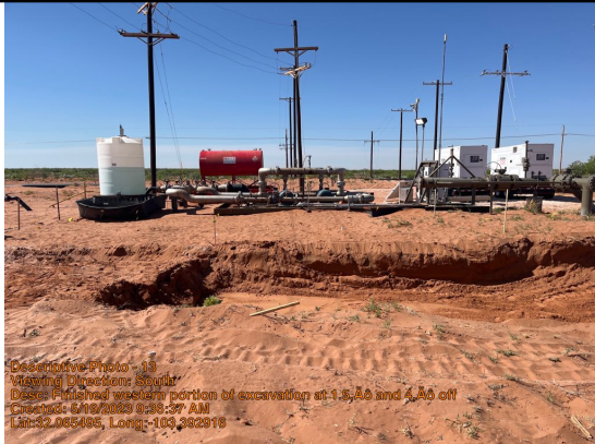
Finished western portion of excavation at 1.5' and 4' off pad.
