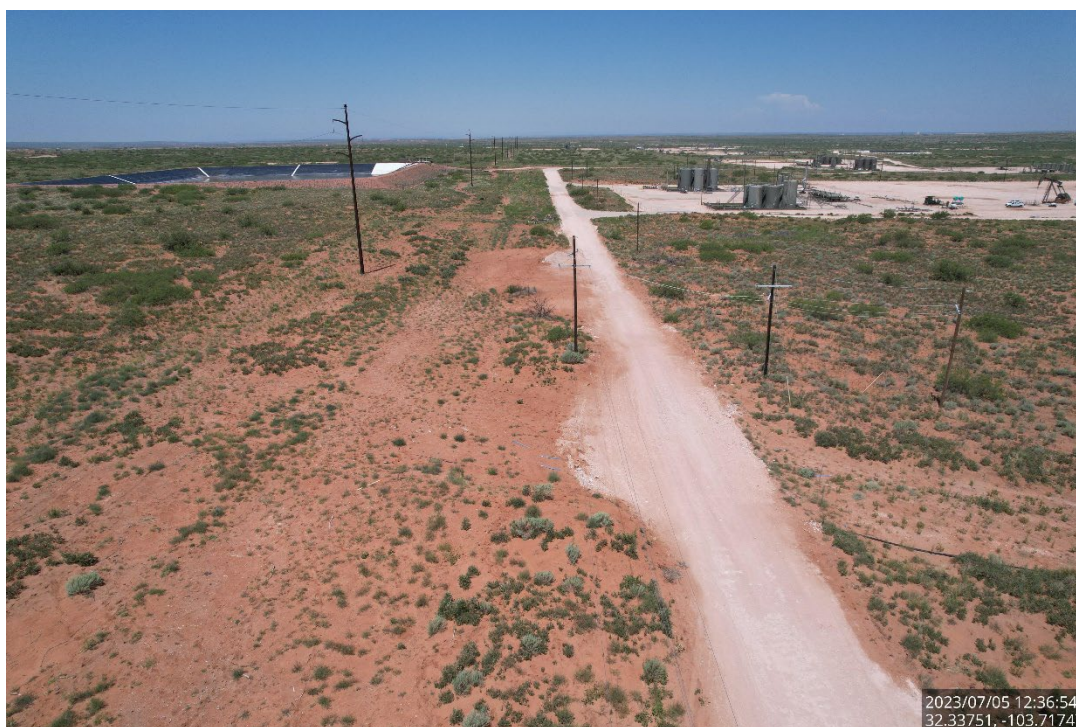
Backfilled and seeded excavation areas, July 5, 2023
