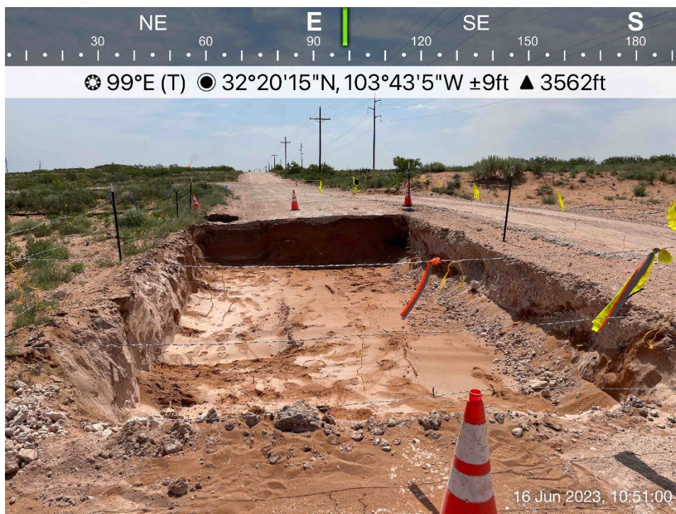
Remaining excavated area viewing east, June 16, 2023
