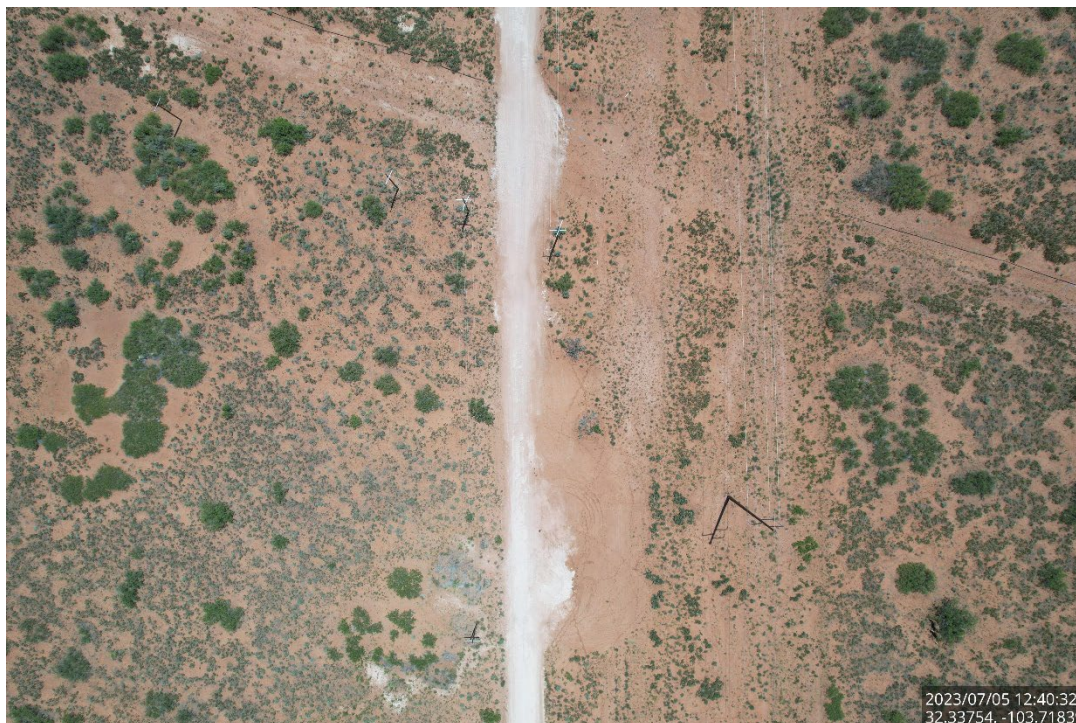
Backfilled and seeded excavation areas, July 5, 2023
