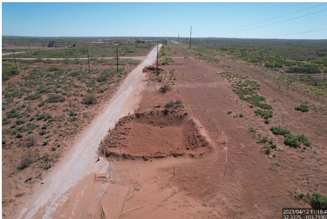
Aerial view of excavated areas, April 12, 2023
