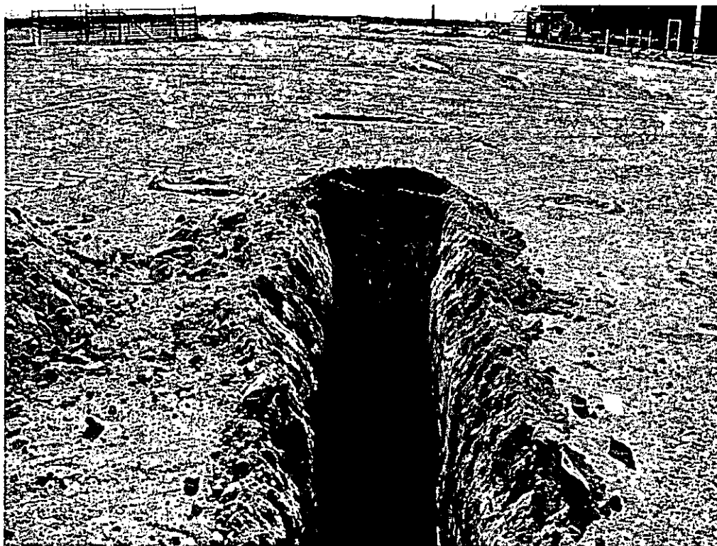
Typical Backhoe Trench
