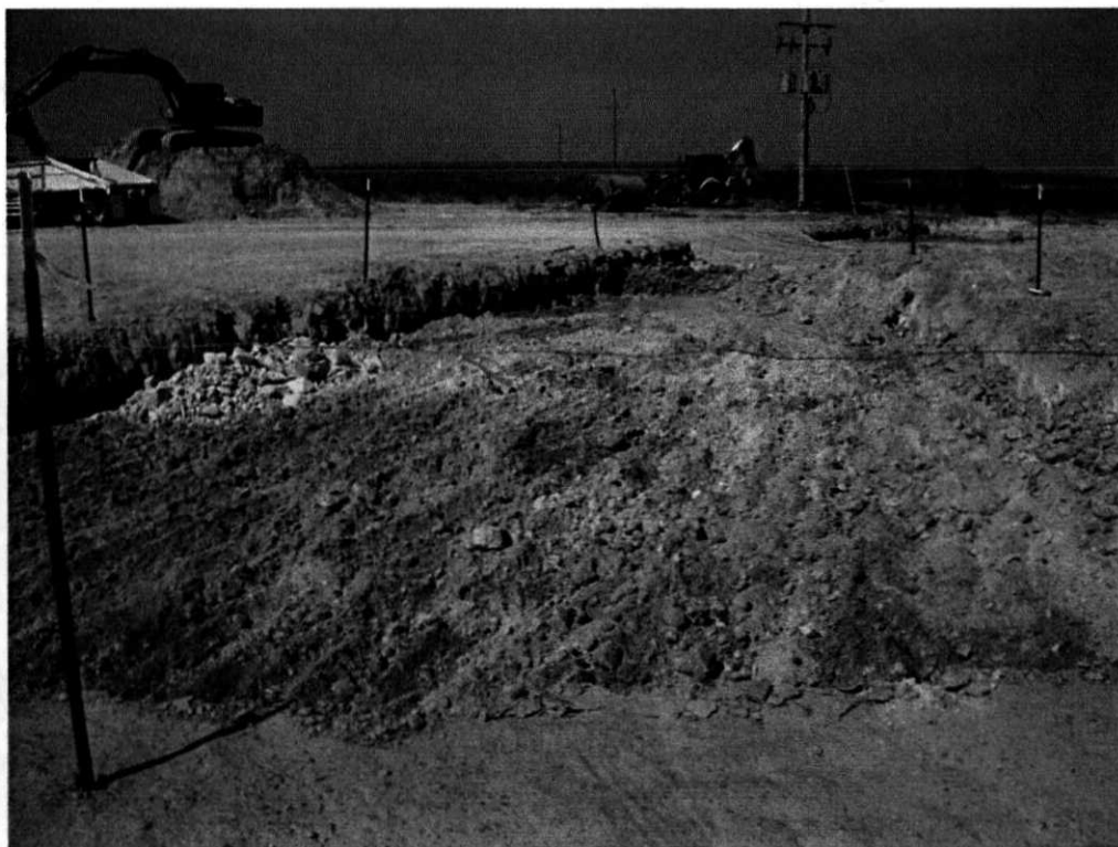
View North – Excavation area of AH-5
