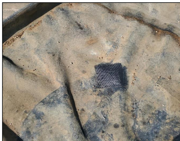
Photograph: 4 Date: 8/4/2023 Description: Patched liner View: South
