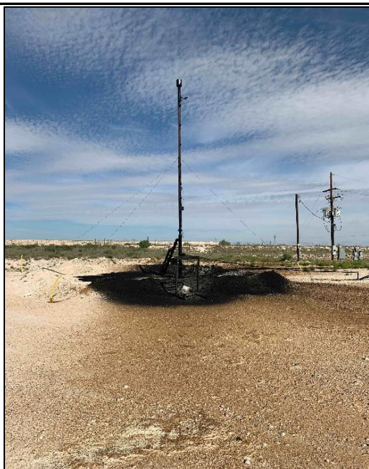
Photograph: 1 Date: 6/11/2023 Description: Initial release discovery View: North
