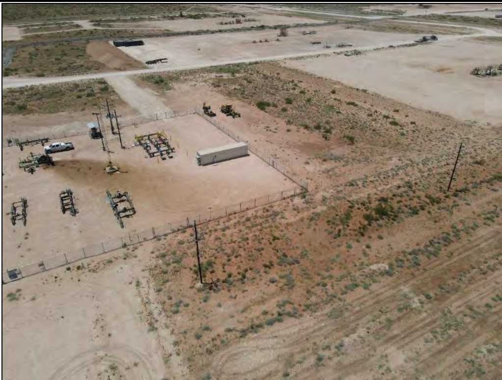
PHOTO 4: View of the impacted area facing southwest. 7/19/23
