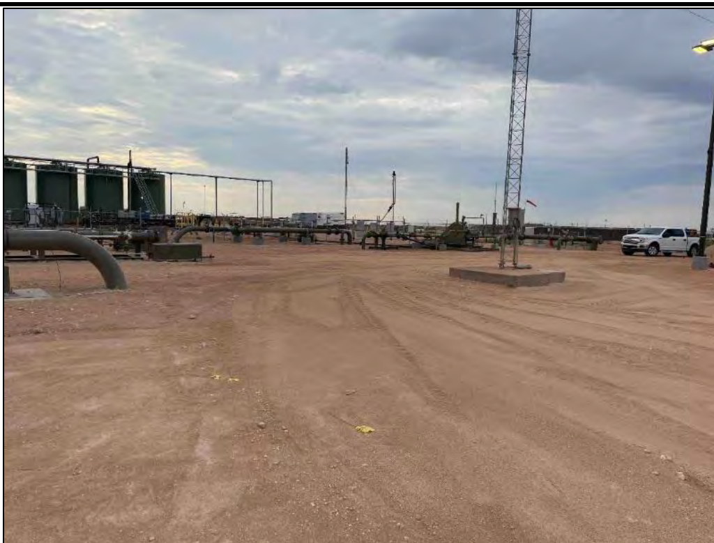
PHOTO 12: View of the remediated area facing southeast. 8/28/23
