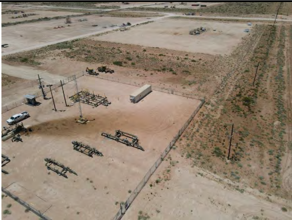
PHOTO 2: View of the impacted area facing west. 7/19/23
