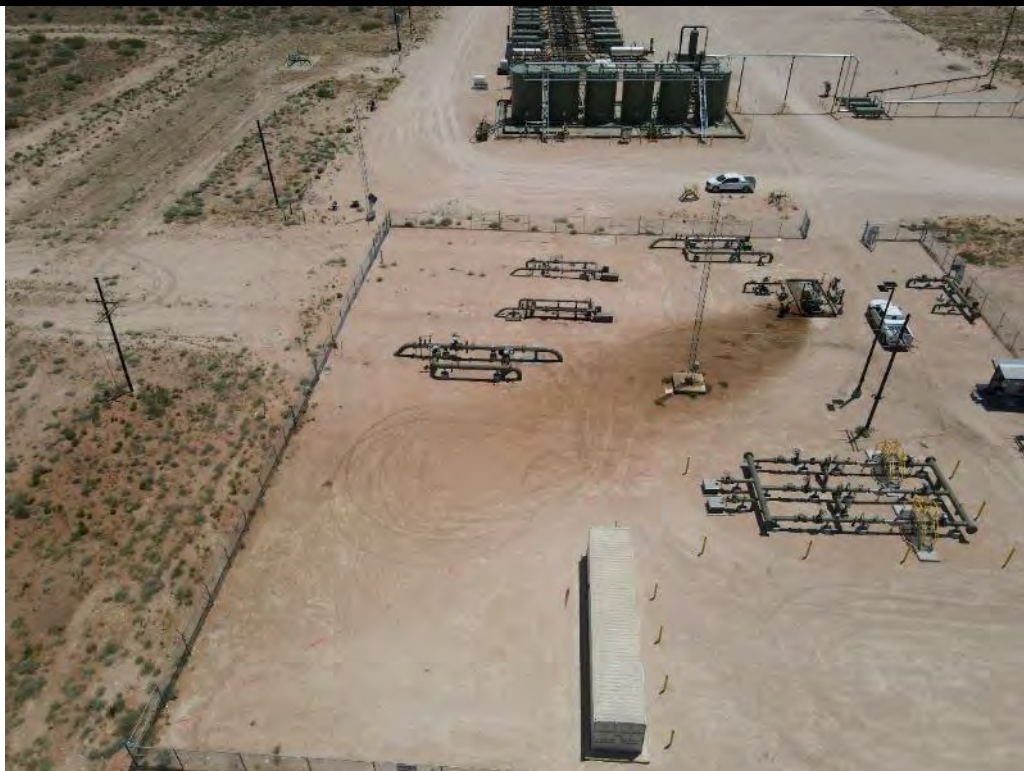
PHOTO 1: View of the impacted area facing west 7/19/23
