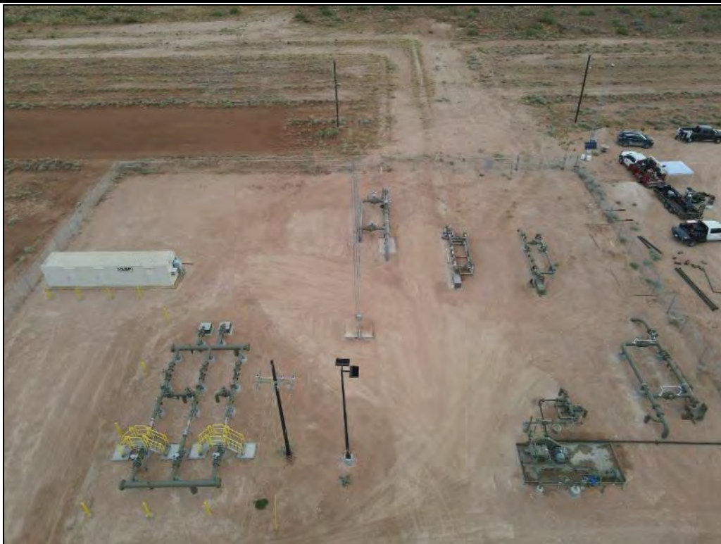
PHOTO 9: View of the remediated area facing north. 8/28/23
