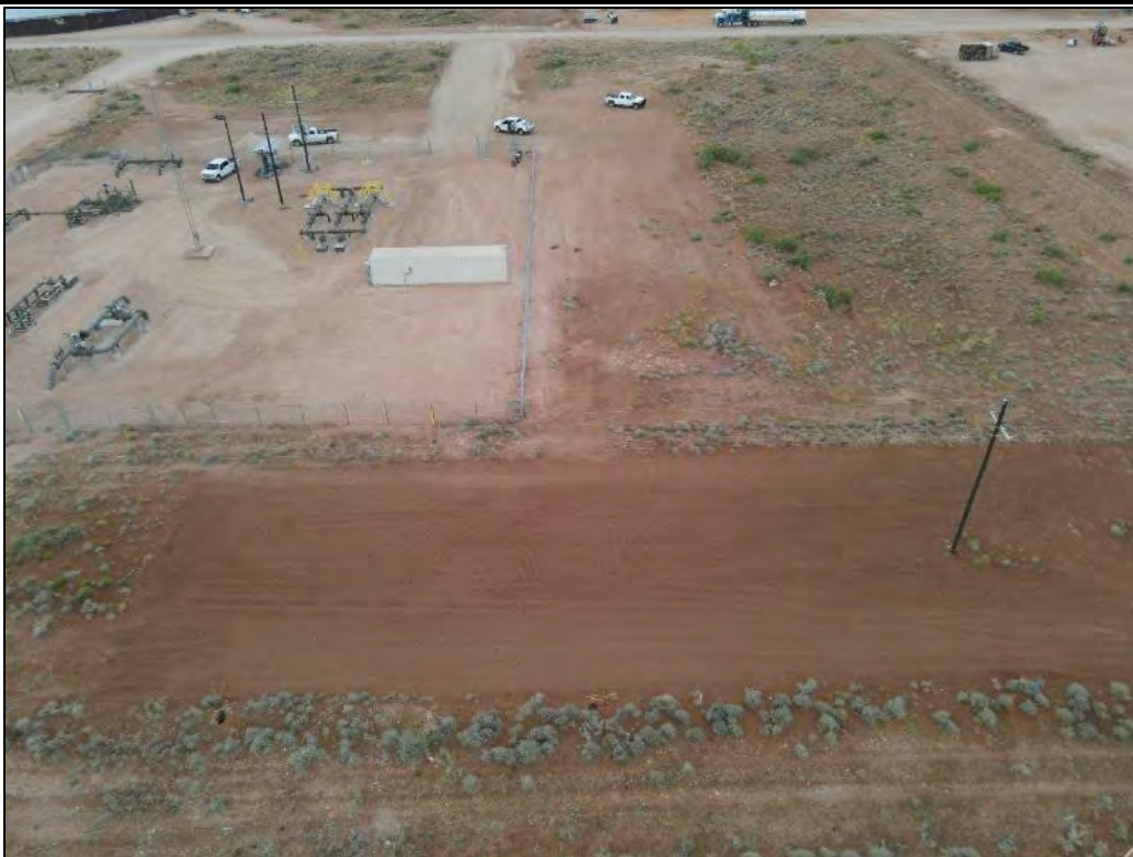
PHOTO 8: View of the remediated area facing south. 8/28/23
