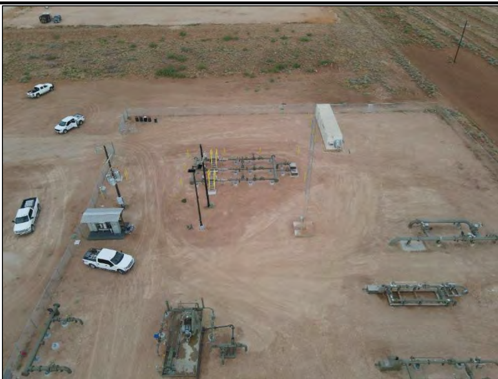
PHOTO 10: View of the remediated area facing west. 8/28/23
