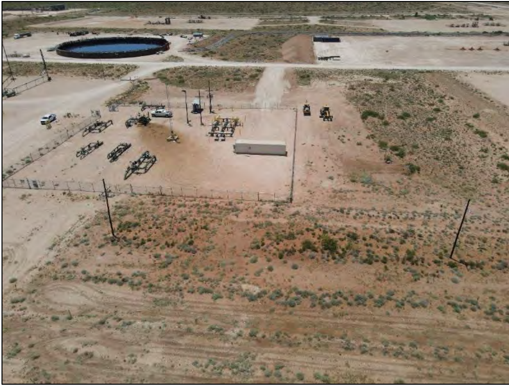
PHOTO 3: View of the impacted area facing southeast. 7/19/23
