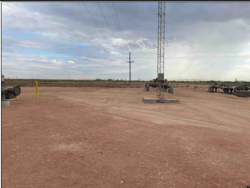
PHOTO 11: View of the remediated area facing north. 8/28/23
