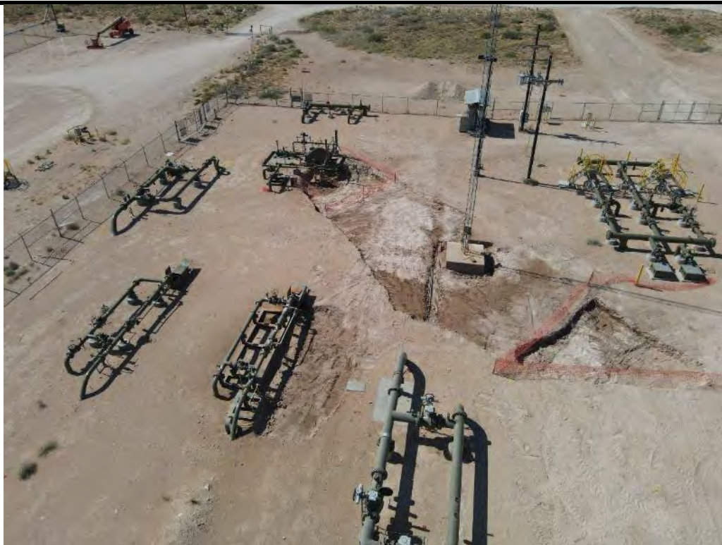
PHOTO 6: View of the excavated area facing south. 8/14/23
