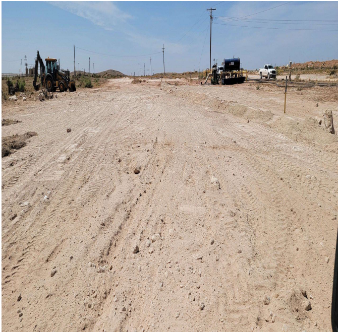
Backfill to grade.
