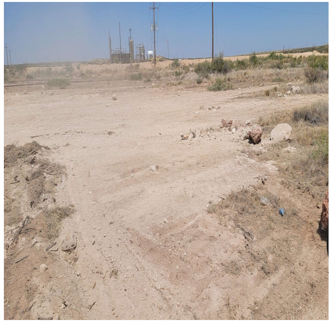
Backfill to grade.
