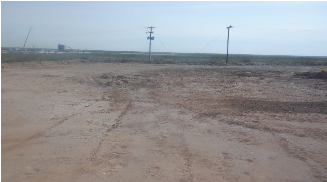
Photo #11 – Excavating & Removing the Containment Berms;
