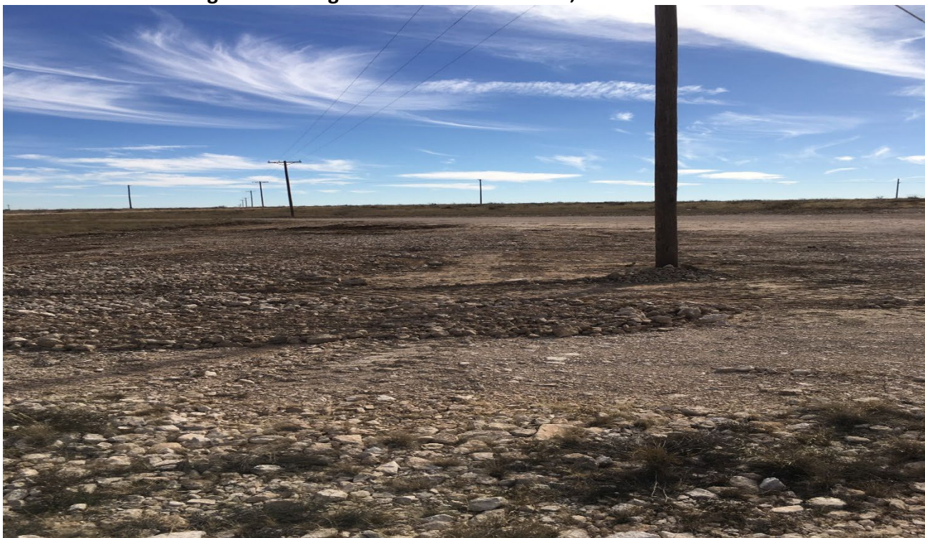
Photo #12 - Excavating & Removing the Containment Berms;
