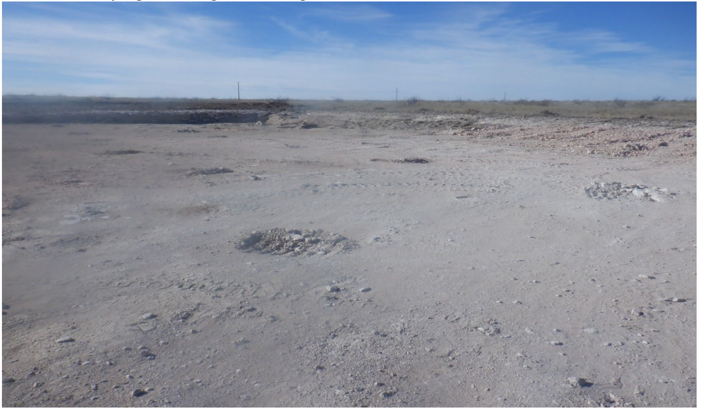
Photo #13 – Sampling, Releveling, & Backfilling
