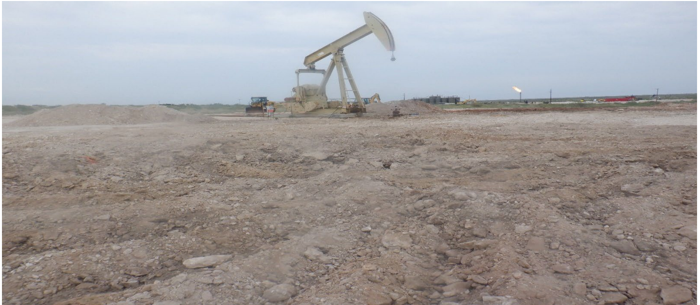
Photo #5 – North Area Excavation
