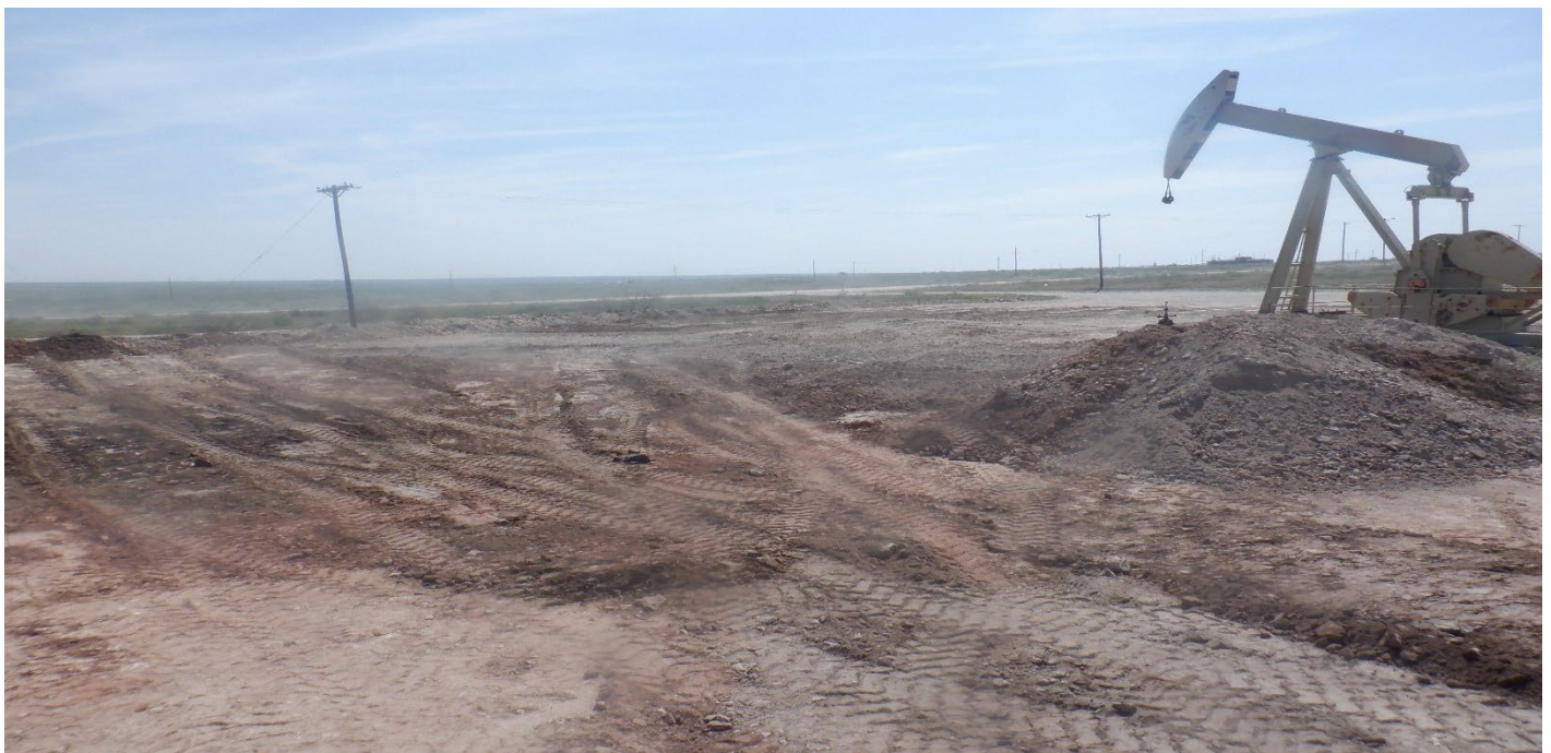
Photo #6 - Contaminated Soil & Excavation
