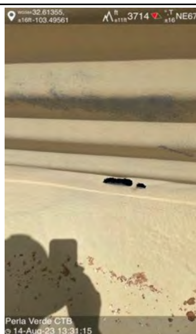
Photograph 2 Date: 8/14/2023 Description: Liner inspection, liner tear on side. View: Northeast
