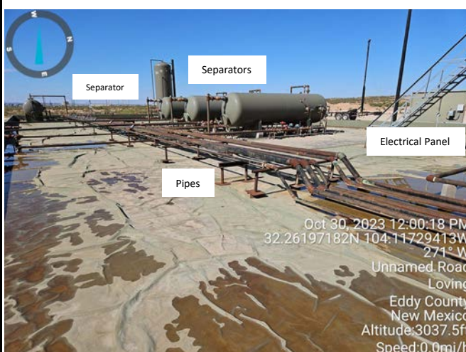
Photograph 4 Date: October 30, 2023 Description: Active equipment inside of lined containment, facing northwest
