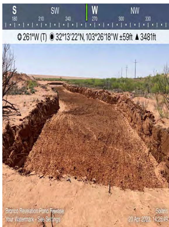
View of Remediation Activities – View West
