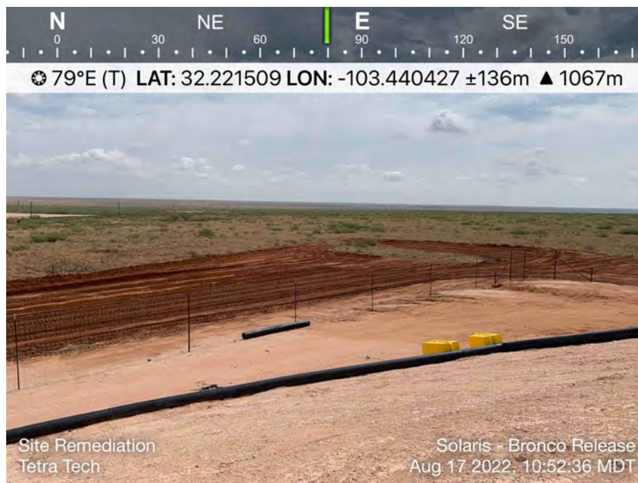
View of Initial Remediation Activities – View East
