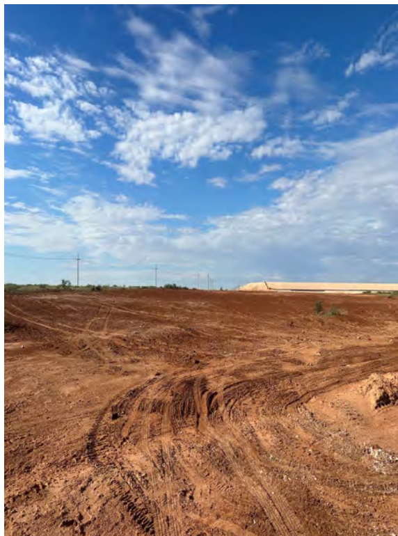
View of Backfilled Area
