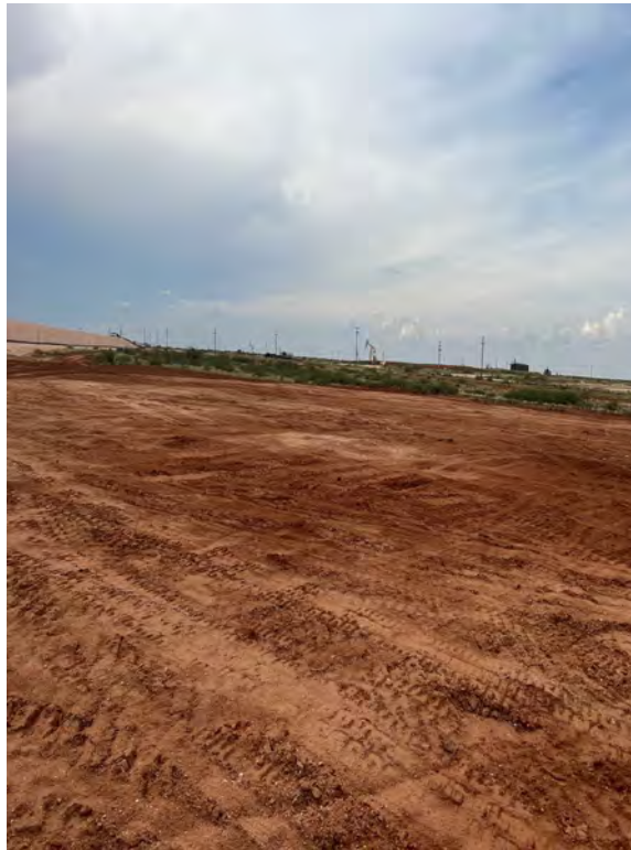
View of Backfilled Area
