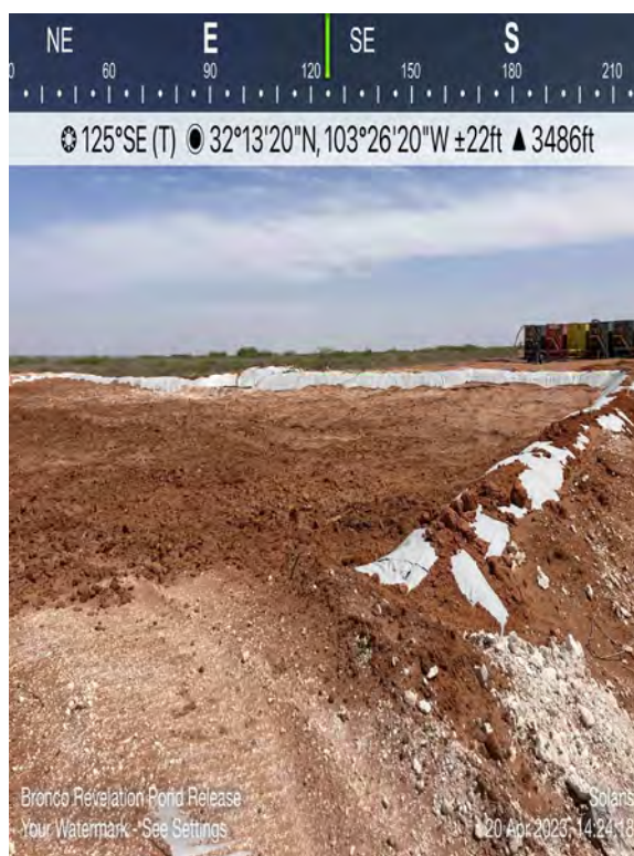
View of Treatment Cell – View Southeast
