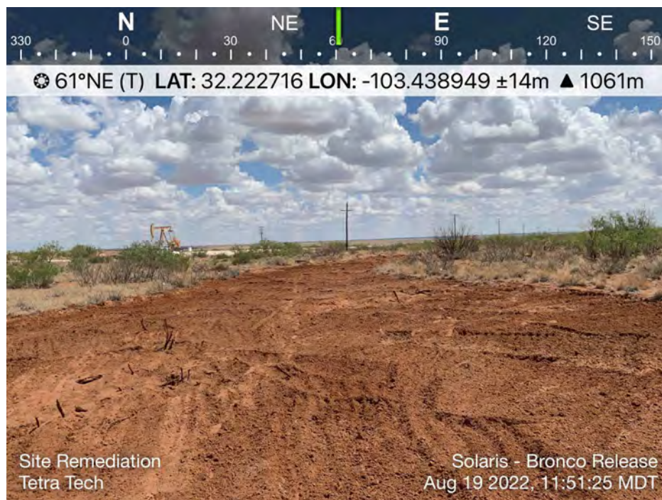
View of Initial Remediation Activities – View Northeast
