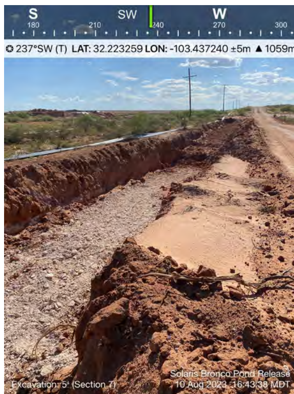
View of Remediation Activities – View Southwest
