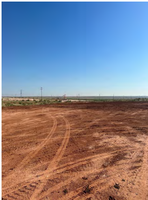
View of Backfilled Area
