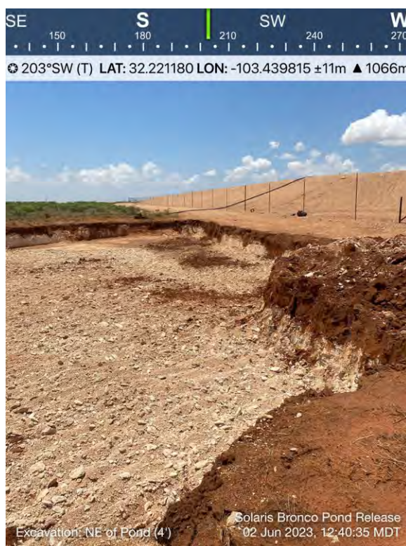
View of Remediation Activities – View Southwest
