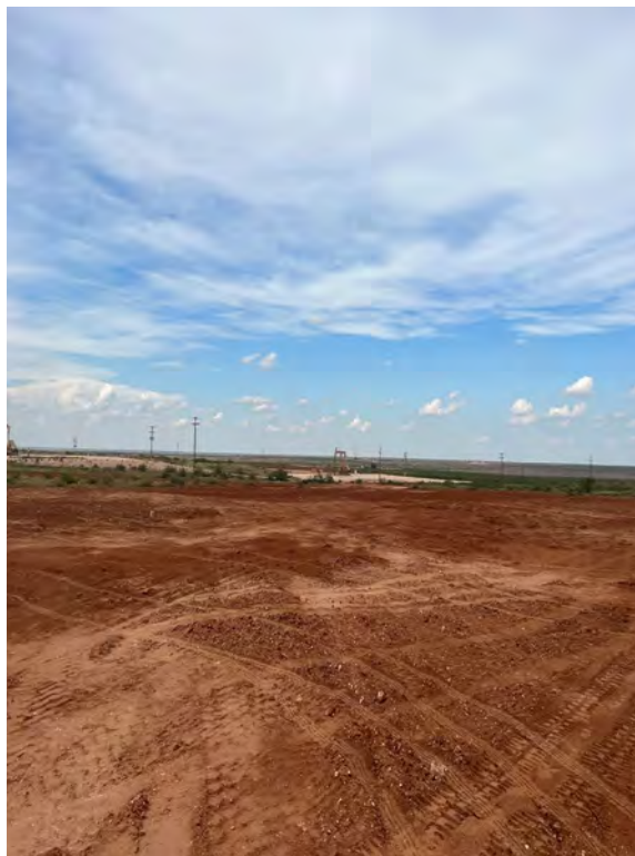
View of Backfilled Area
