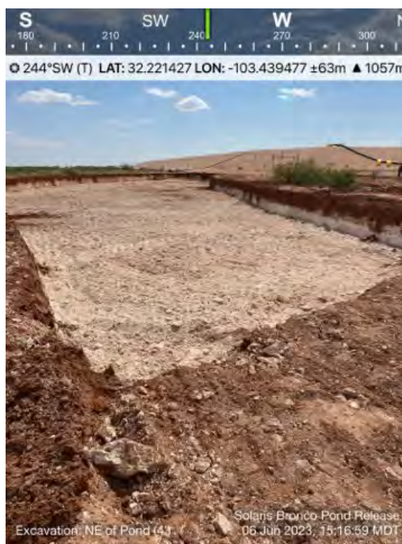
View of Remediation Activities – View Southwest
