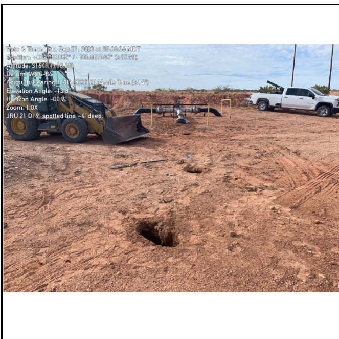
Photograph 2 Date: 9/21/2023 Description: Hydro-vac spotting produced water pipeline View: South
