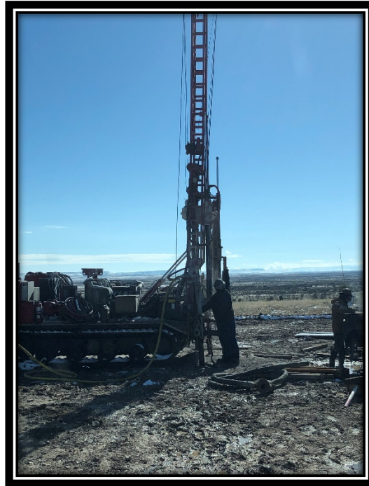
Photo 5: Exploratory Soil Boring (SB-8)
