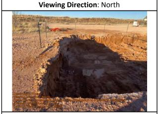
North of pump jack facing north. Excavation to 4 feet bgs completed.
