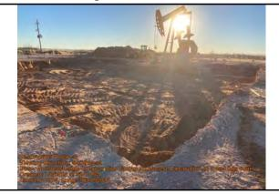
Northeast edge of excavation facing southwest. Excavation to 4 feet bgs completed.
