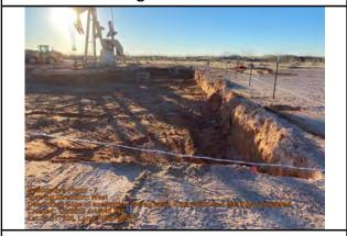
Northeast edge of excavation facing west. Excavation to 4 feet bgs completed.
