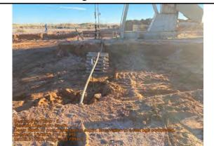
North of pump jack facing south. Excavation to 4 feet bgs completed.
