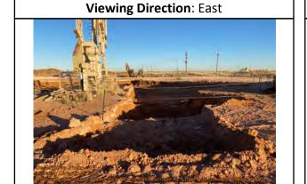
Southwest of pump jack facing east. Scrape to 1 foot bgs on west side completed.
