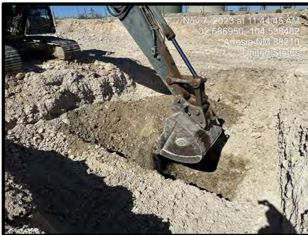
PHOTOGRAPH NO. 3 – A view of the soil removal operations in the area exhibiting discolored soil, hydrocarbon odors, and elevated OVM readings. The view is towards the northwest.
