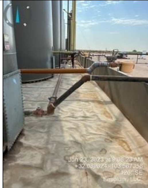
Photograph: 6 Date: 6/23/2023 Description: View of lined containment deemed to be in good condition, facing southeast
