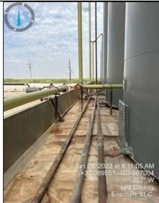
Photograph: 8 Date: 6/23/2023 Description: View of lined containment deemed to be in good condition, facing west
