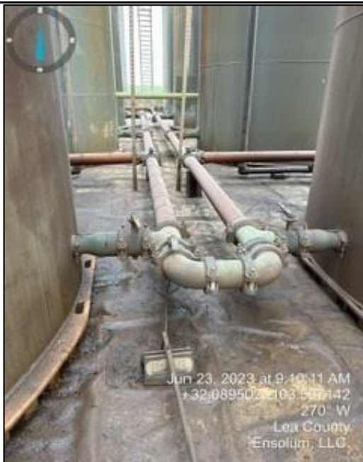
Photograph: 7 Date: 6/23/2023 Description: View of lined containment deemed to be in good condition, facing west
