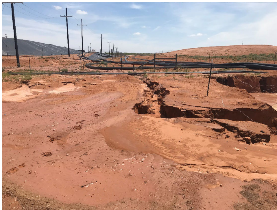
Completed excavation on May 3, 2023, viewing to the north (32.39055, -103.72305).
