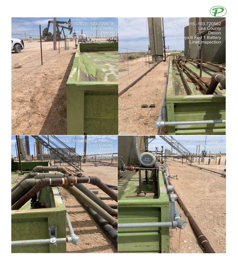
The Liner shows evidence of discoloration and sun deterioration, Liner does have the integrity to retain fluids
