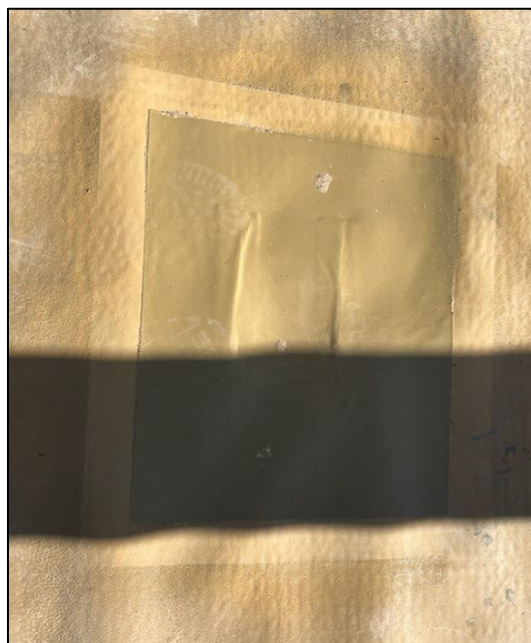
Photograph: 6 Date: 3/1/2024 Description: Patched liner. View: N/A
