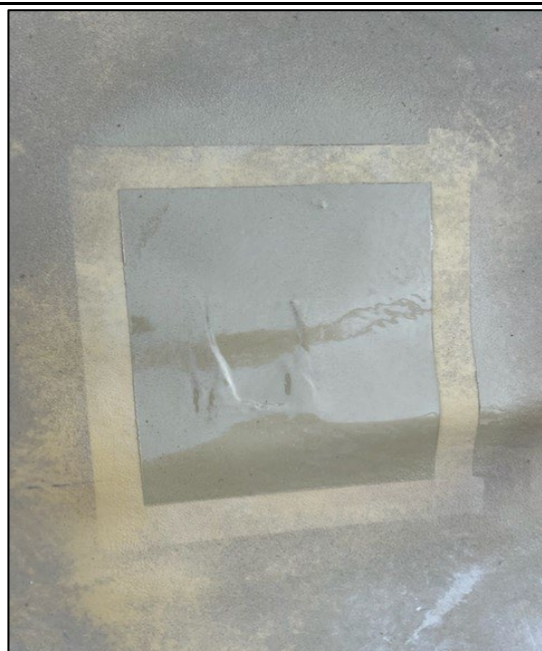
Photograph: 7 Date: 3/1/2024 Description: Patched liner. View: N/A
