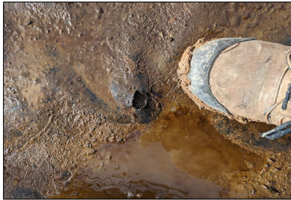
Photograph: 3 Date: 1/29/2024 Description: Liner Holer View: NA
