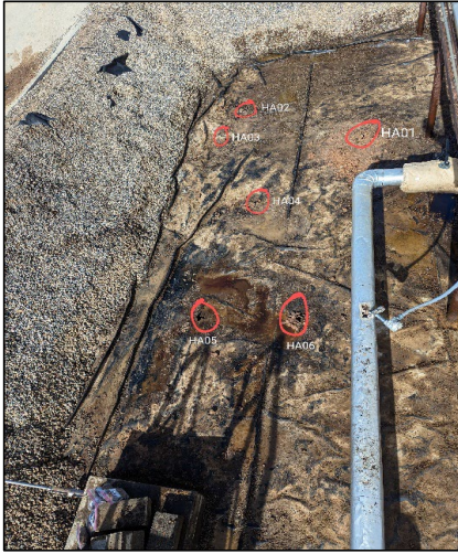
Photograph: 1 Date: 1/29/2024 Description: Liner Holes/Sampling Locations View: North
