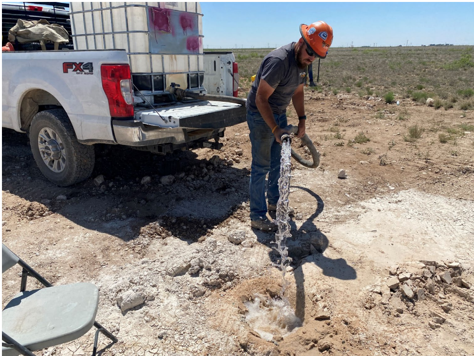
Photograph 8: Adding water to backfilled borings in order to hydrate the bentonite chips
