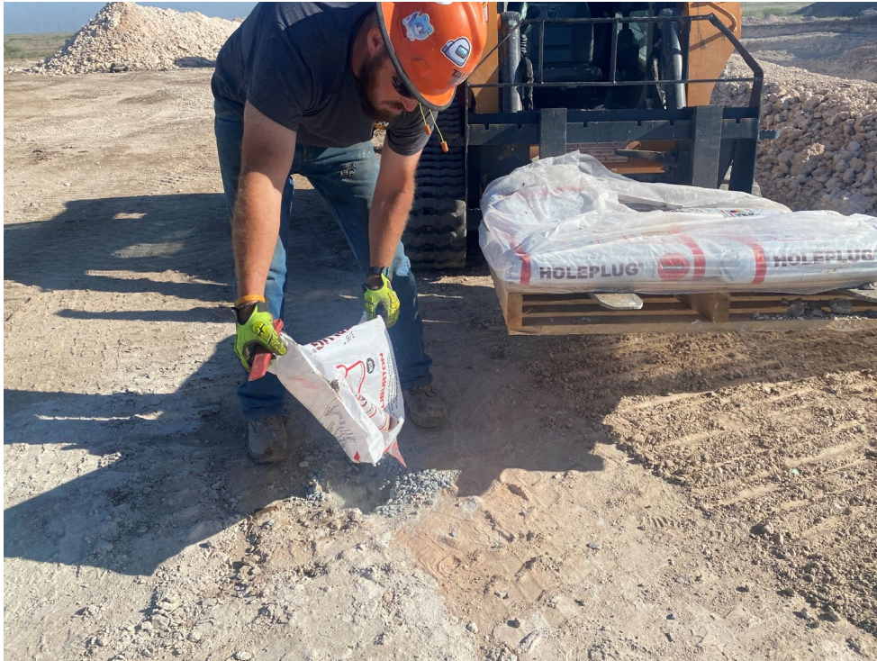
Photograph 7: Backfilling borings with 3/8" Hole Plug bentonite chips
