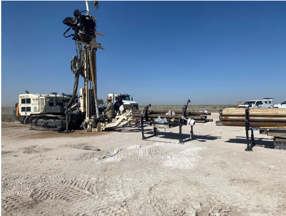
Photograph 3: Drilling rods and casing staged near rig during drilling
