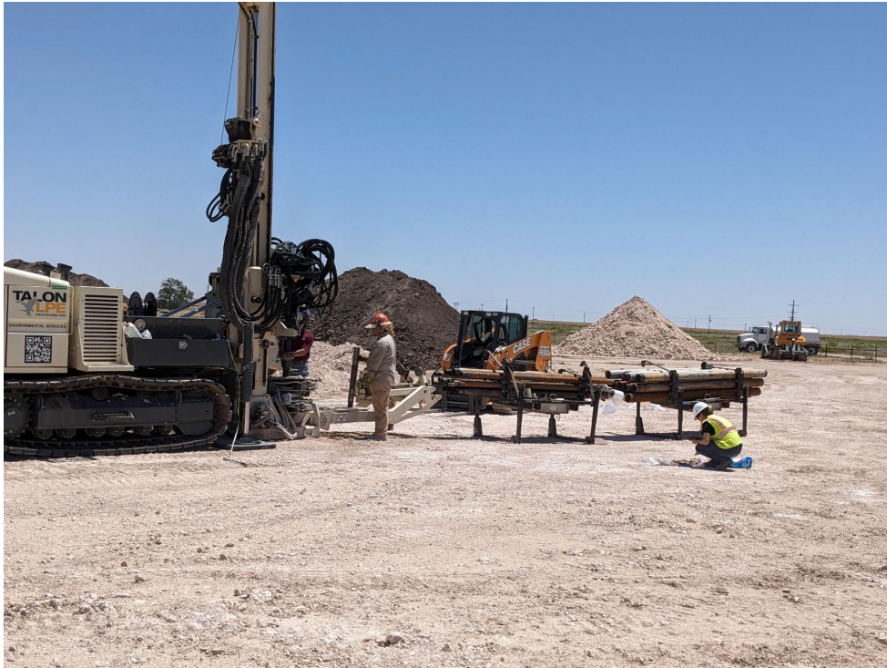
Photograph 4: INTERA geologist collecting core samples for field screening and borehole logging
