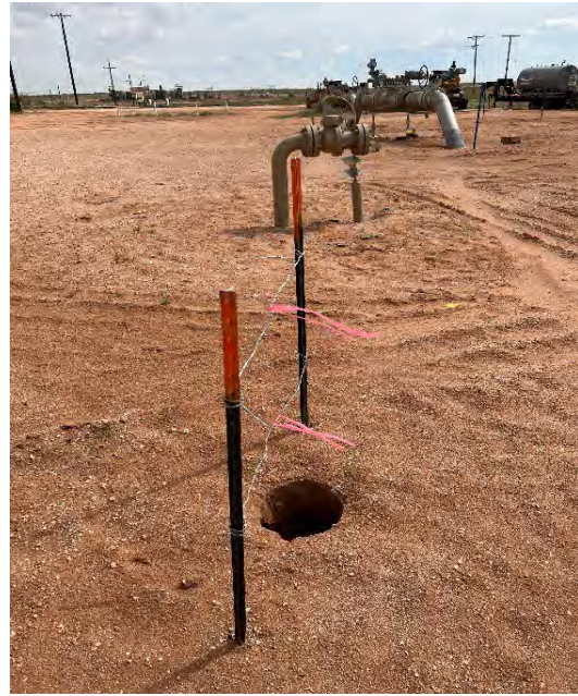
Photograph: 2 Date: 8/1/2022 Description: Pothole delineation BH05. View: South
