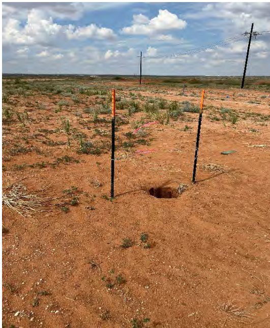
Photograph: 3 Date: 8/1/2022 Description: Pothole delineation BH02. View: Northeast
