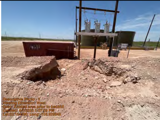
Eroded area on west edge of pad
