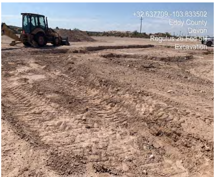
Excavation East side
