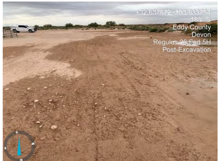
Backfill West side (Rainwater)
