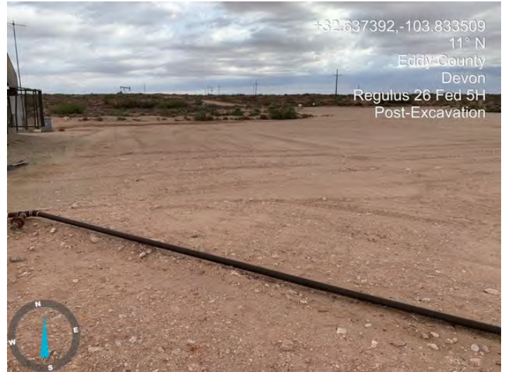
Backfill East side
