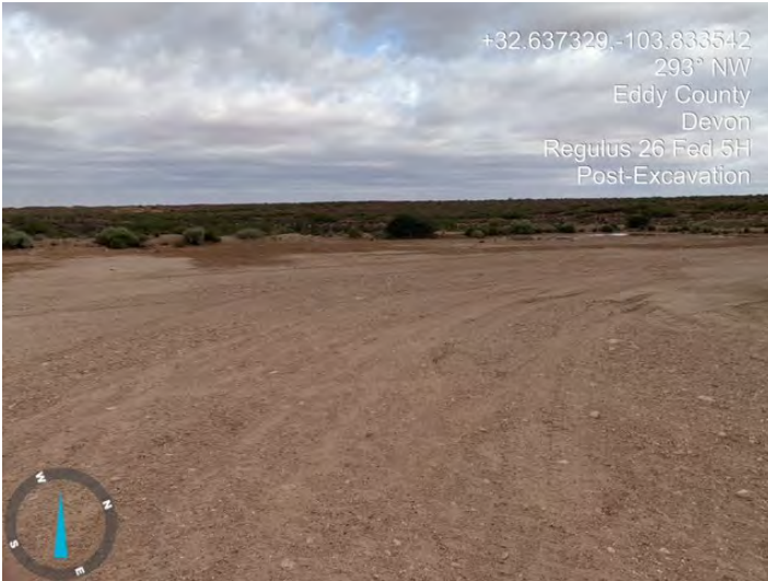
Backfill West side
