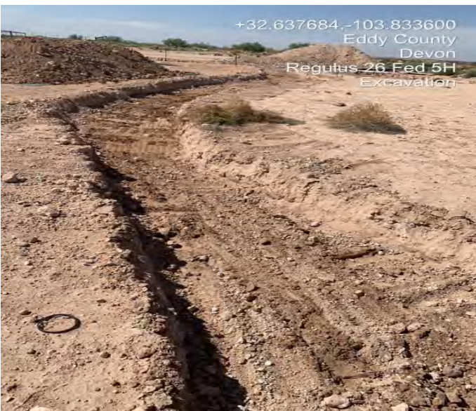
Excavation West side
