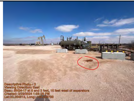
BH24-17 at 0 and 2 feet, 15 feet west of separators
