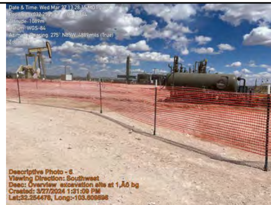
Overview excavation site at 1' bgs. NE part
