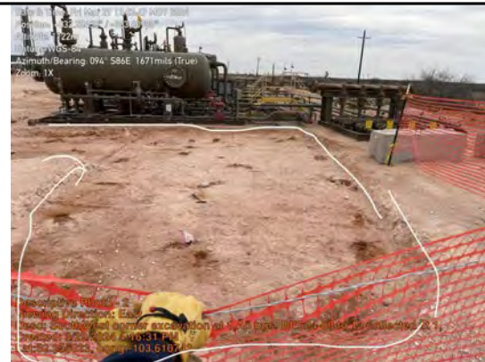
SouthWest corner excavation at 1' bgs. BES24-09 to 12 collected at 1'.
