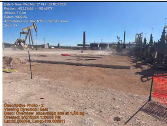
Overview excavation site at 1' bgs
