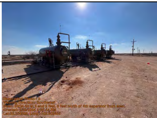
BH24-20 at 0 and 2 feet. 6 feet north of 4th separator from west.
