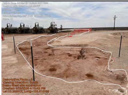
West site excavation at 1' bgs
