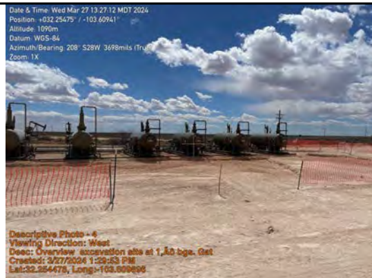
Overview excavation site at 1' bgs. Gate
