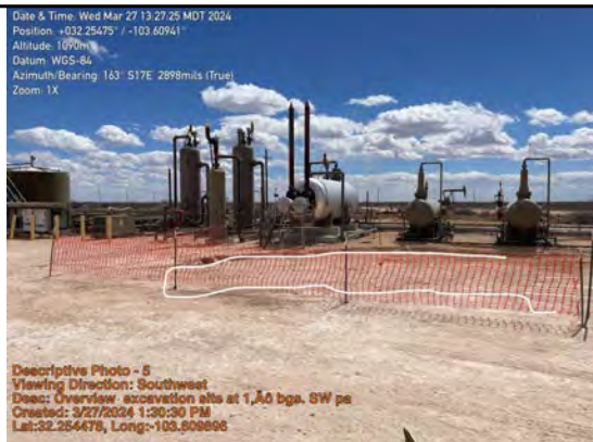
Overview excavation site at 1' bgs. SW part
