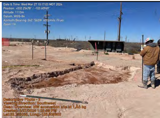
Overview NW excavation site at 1' bgs
