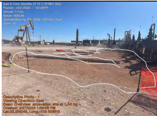
Overview excavation site at 1' bgs
