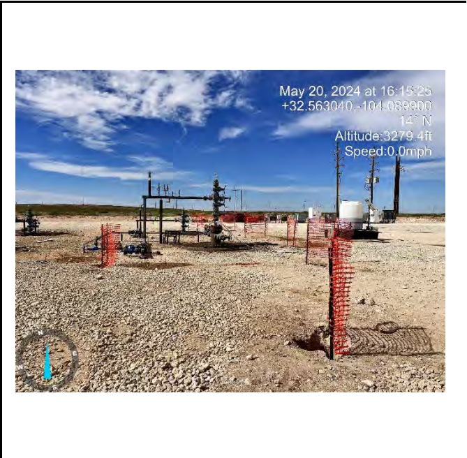
Photograph 6 Date: 5/20/2024 Description: Hydrovac View: North
