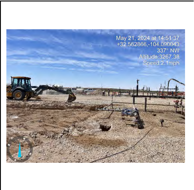
Photograph 8 Date: 5/21/2024 Description: Excavation View: North
