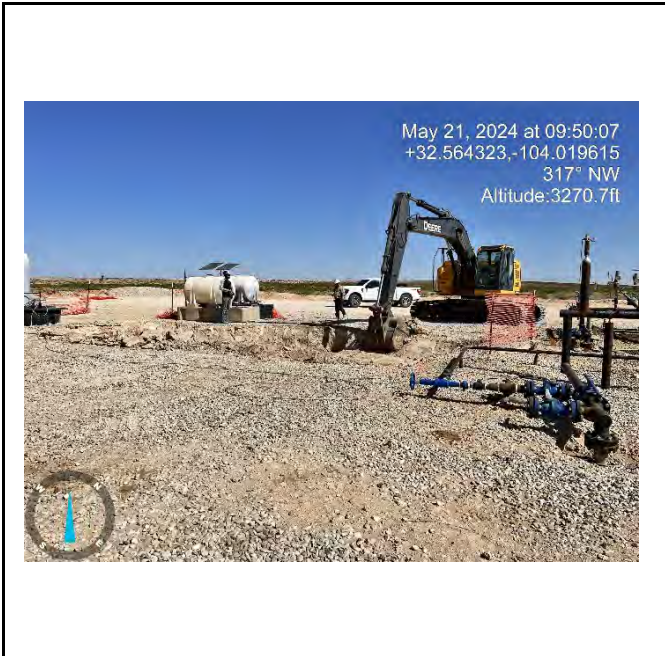
Photograph 7 Date: 5/21/2024 Description: Excavation View: Northwest
