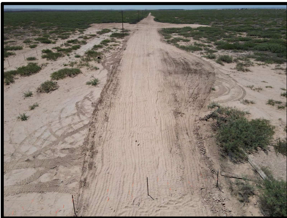
PHOTOGRAPH NO. 4 – A view of the Site upon completion of the backfill and tilling operations. The view is towards the south.
